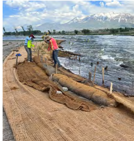
Crews reinforce delta streambank during high flows
