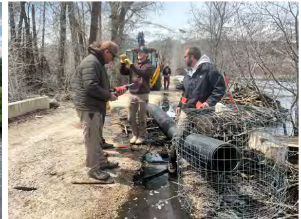
Installing a pond leveler to help prevent road flooding
