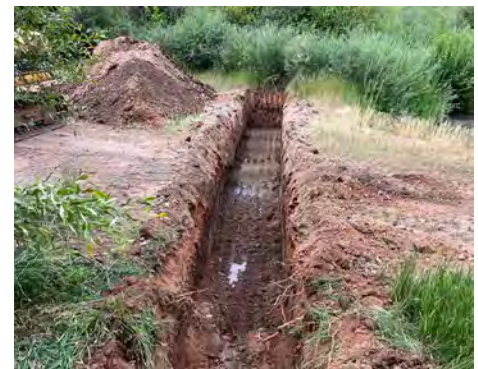
Cutoff wall created to control eroding bank
