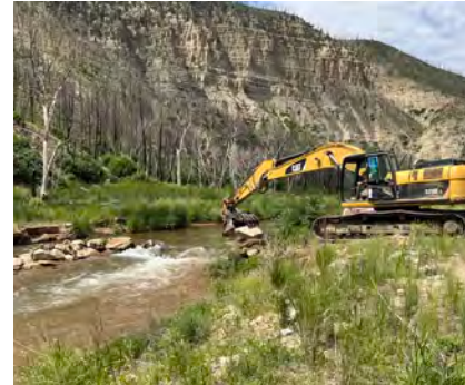
Work on Strawberry River cross vanes, man-made fish habitat structures that also stabilize streambanks
