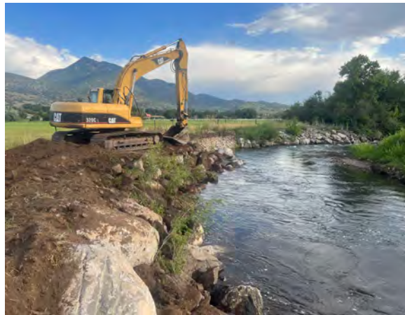
Construction to stabilize PRRP river bend
