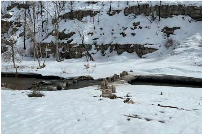
Post Assisted Log Structure constructed to catch instream debris
