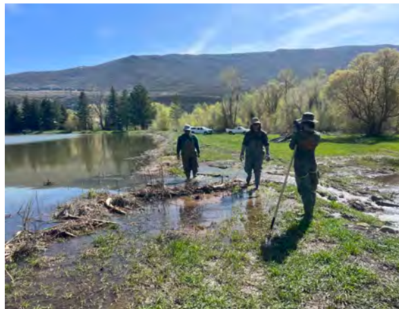
Condie Pond outlet maintenance and clearing
