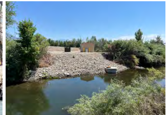
Structure built to house original channel aeration system
