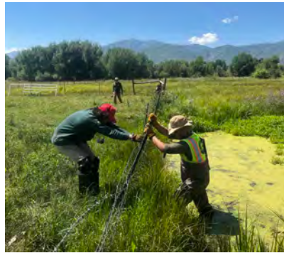
Repairing PRRP boundary fence
