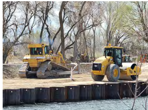
Construction of Provo River Delta diversion structure
