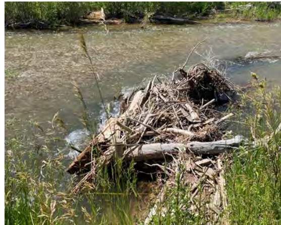
Post-assisted log structure after 2023 spring runoff
