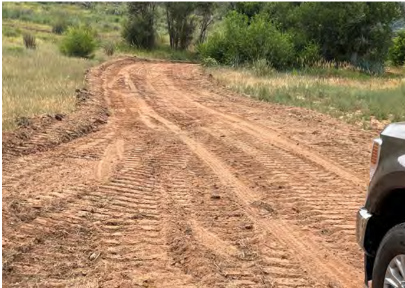
Newly constructed road segment
