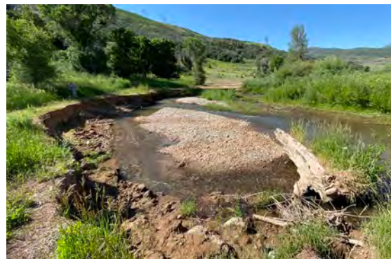
Bank area in need of stabilization
