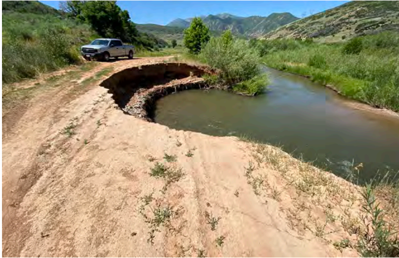
Access road in need of re-routing
