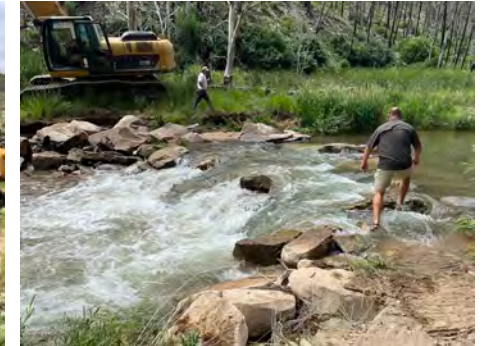
Work on Strawberry River cross vanes, man-made fish habitat structures that also stabilize streambanks
