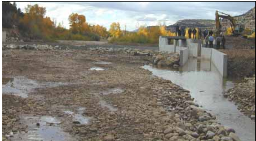
Newly constructed WPPB diversion on the Duchesne River
