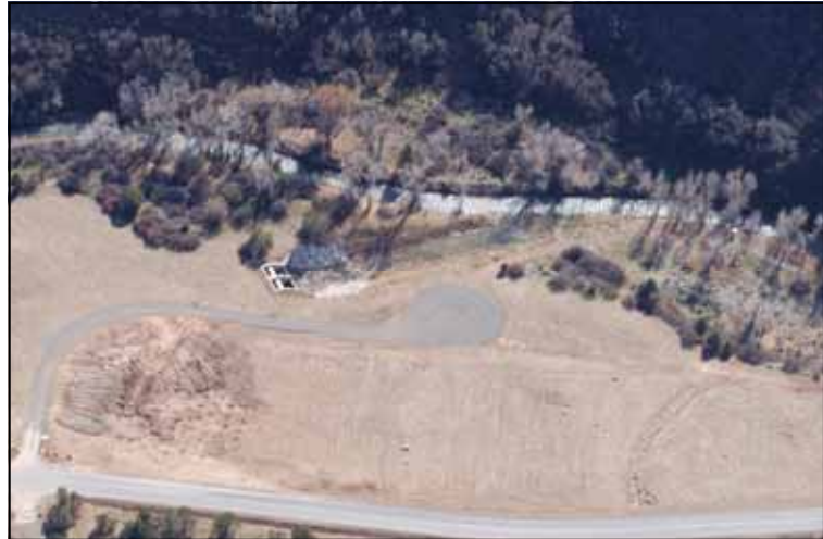
The Diamond Fork Outlet (left/center) is used to make supplemental instream flow releases into Diamond Fork Creek; the facility also will release flows in excess of the Diamond Fork Pipeline capacity (560 cfs), into Diamond Fork Creek. The Diamond Fork Group Campground will be constructed on this site in 2006.
