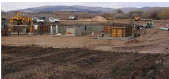
Construction at Whiterocks State Fish Hatchery, September 2005
