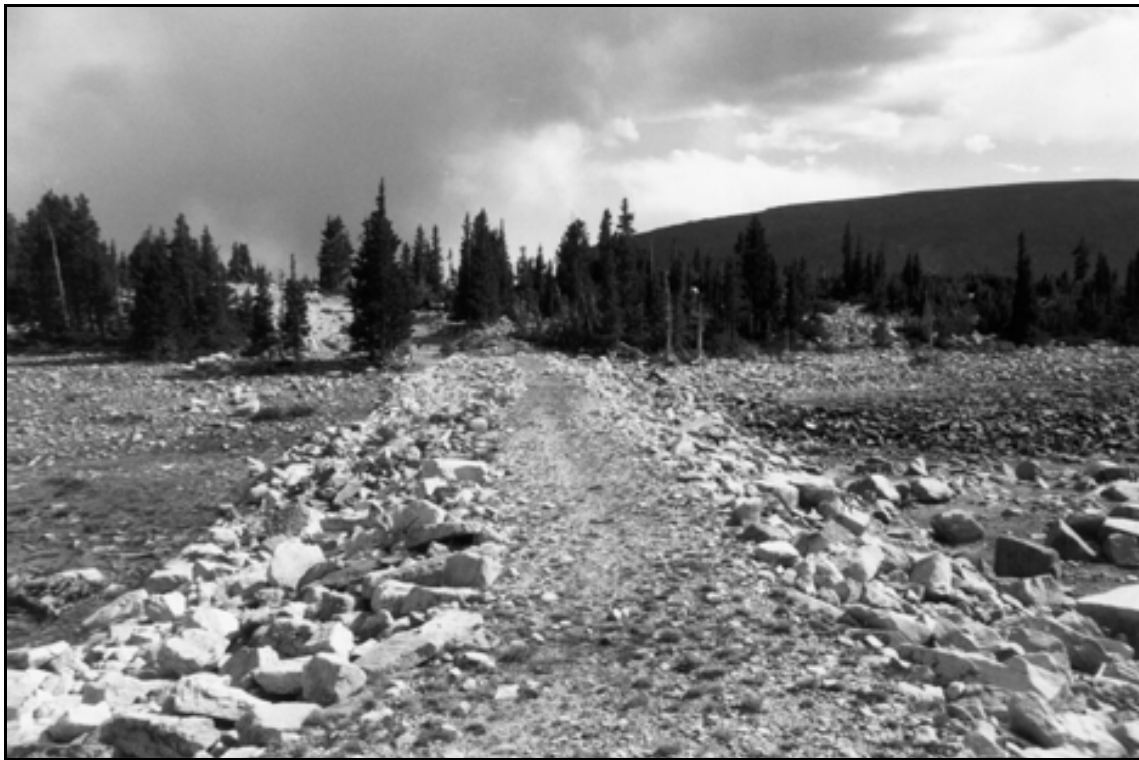
HAER UT-42-E. Drift Lake Dam. Overview of dam surface; view to the south-southeast.
