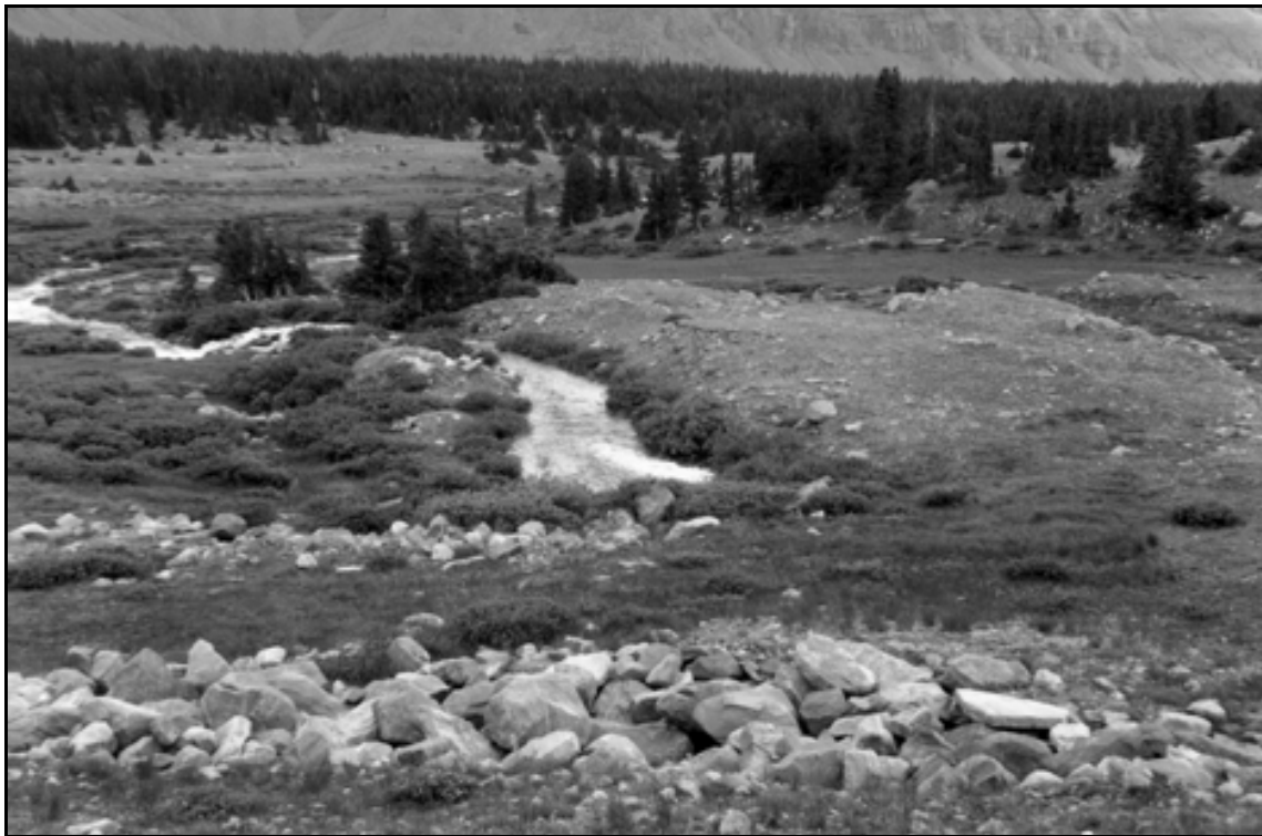
HAER UT-42-F. East Timothy Lake Dam. Overview from dam showing outlet channel; view to the southeast.
