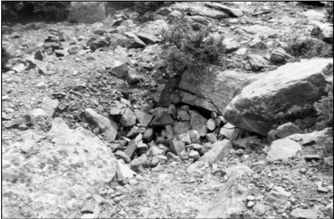
HAER UT-42-G. Farmers Lake Tunnel. Overview of depression east of the tunnel upstream outlet; close-up view.
