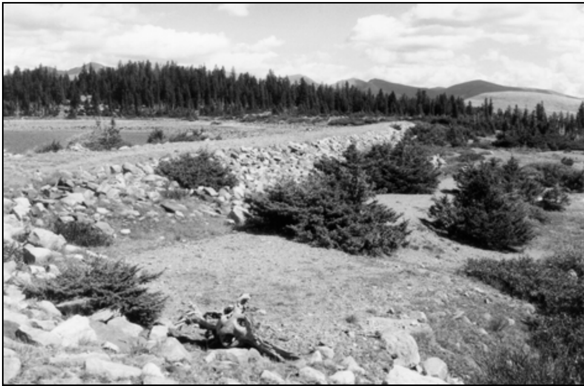
HAER UT-42-H. Five Point Lake Dam. Dam overview, showing ramp from barrow area; view to the northeast.
