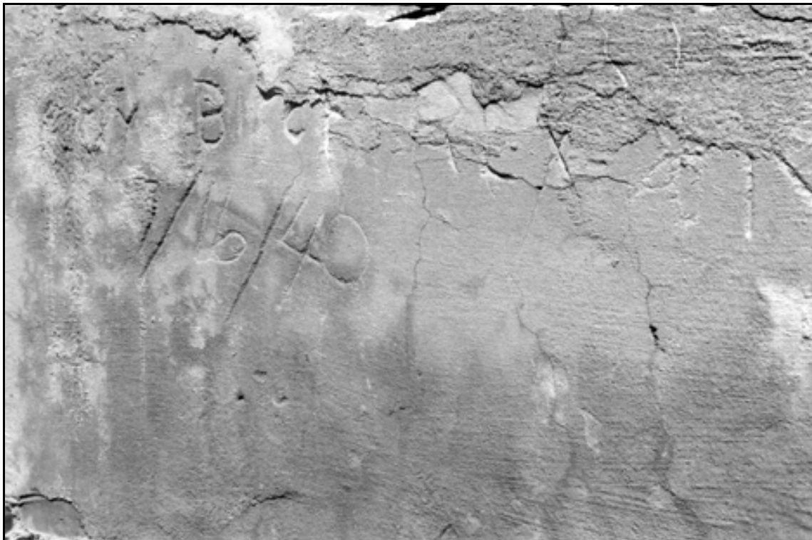
HAER UT-42-H. Five Point Lake Dam. Detail of south face of control box showing inscriptions; close-up view.
