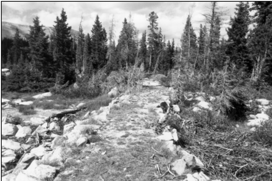
HAER UT-42-A. Bluebell Lake Dam. Overview of dam surface at south end of Dam #2; view to the south-southeast.
