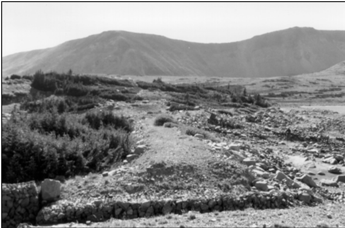
HAER UT-42-L. Superior Lake Dam. Overview of dam showing spillway channel in foreground; view to the southwest.
