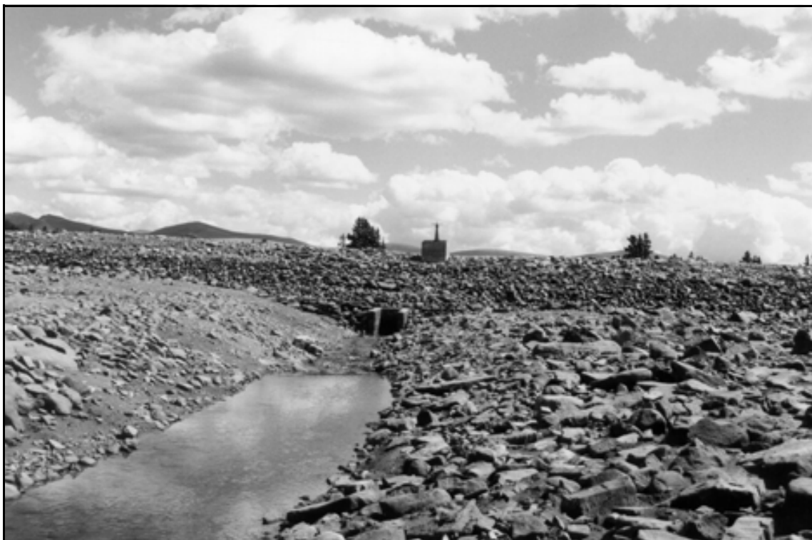
HAER UT-42-H. Five Point Lake Dam. Overview of dam showing upstream outlet and control box; view from reservoir to the east.
