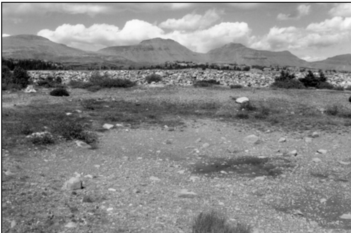
HAER UT-42-H. Five Point Lake Dam. Dam overview from barrow pit; view to the north.
