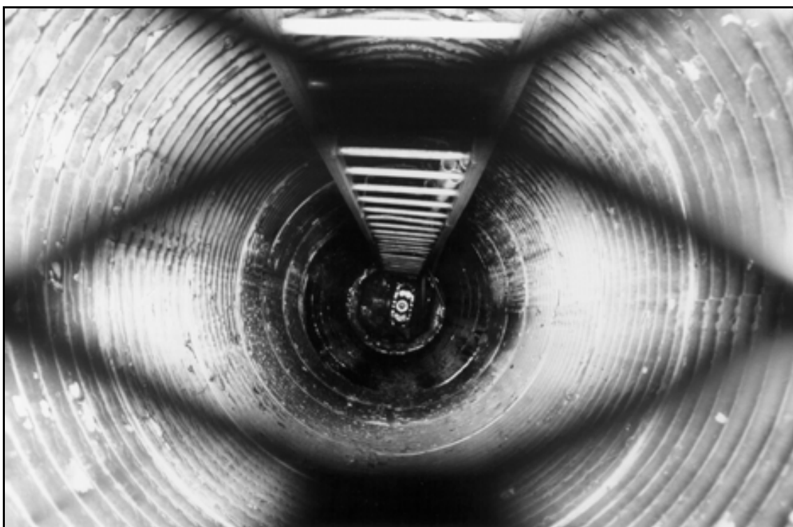
HAER UT-42-F. East Timothy Lake Dam. Looking down culvert shaft toward control gate; close-up view.
