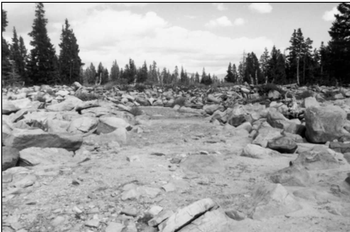
HAER UT-42-A. Bluebell Lake Dam. Overview of Ramp #2 from barrow area to Dam #2; view to the northeast.
