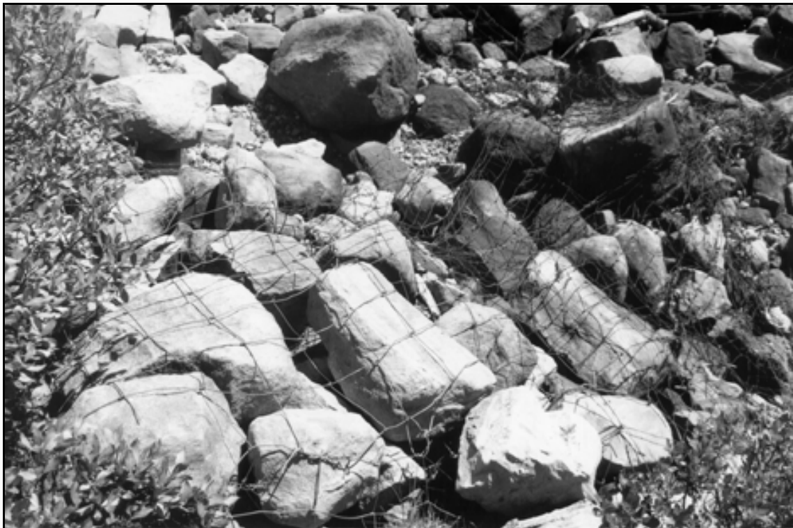
HAER UT-42-H. Five Point Lake Dam. Detail of reinforced area of spillway; view to the south.
