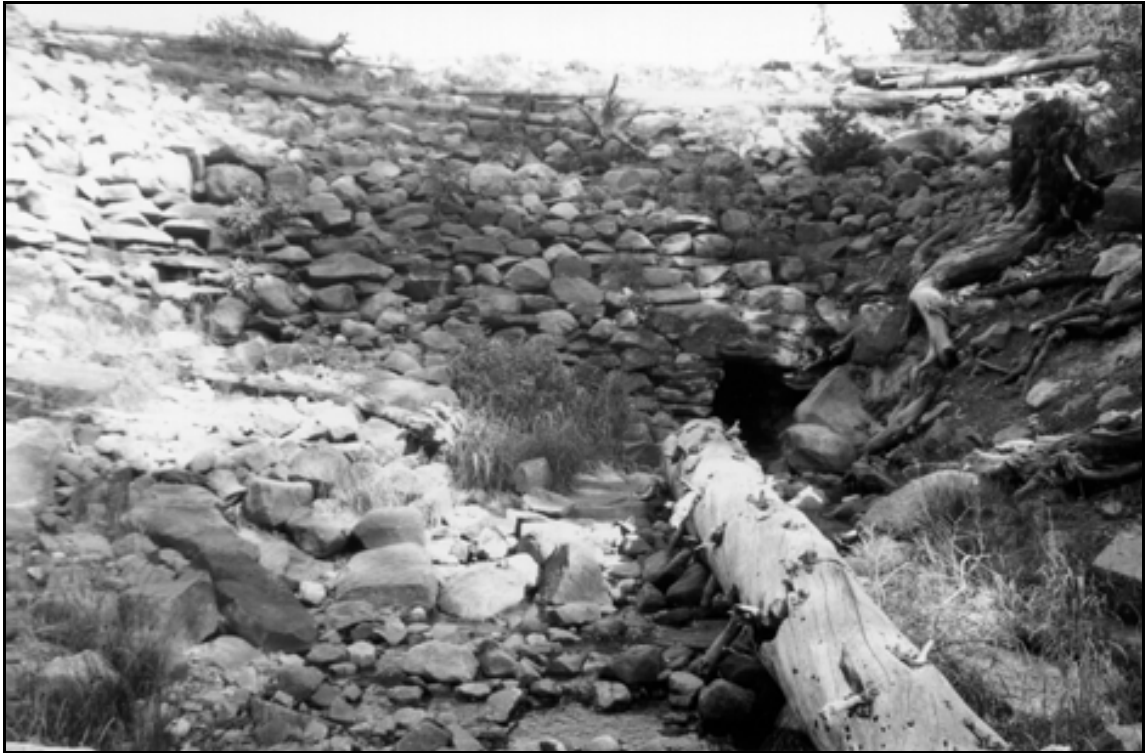
HAER UT-42-D. Deer Lake Dam. Overview of downstream face of dam showing outlet channel; view to the north.
