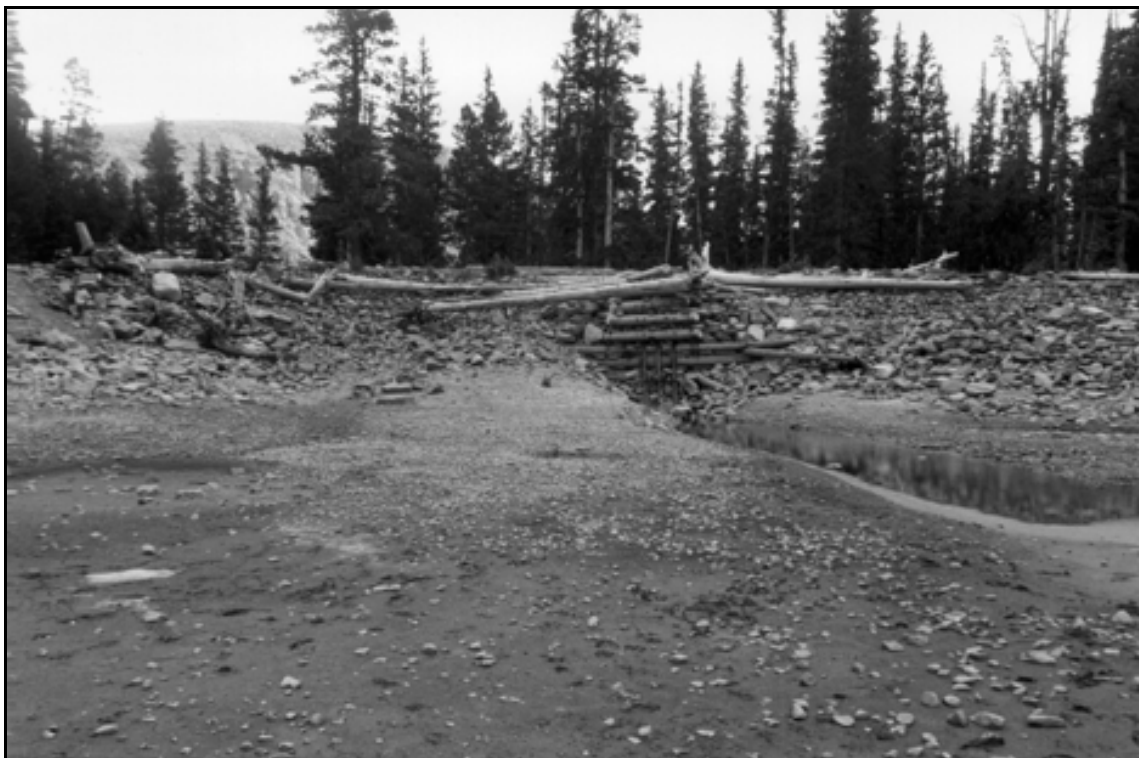
HAER UT-42-D. Deer Lake Dam. View showing profile of the dam from the low water mark; view to the south.
