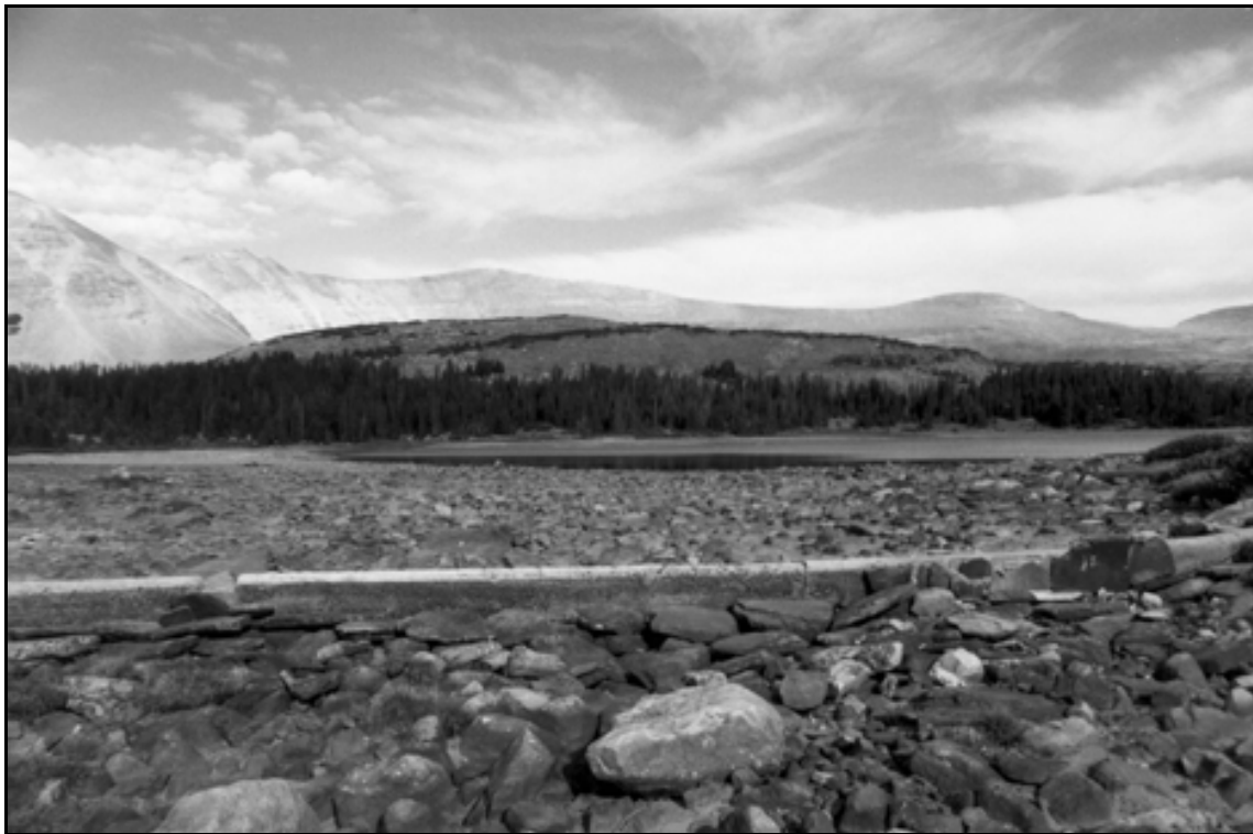
HAER UT-42-H. Five Point Lake Dam. Overview showing upstream view of curb and overflow spillway, lake in background; view to the northwest.
