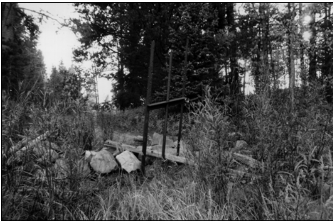
HAER UT-42-N. Water Lily Lake Dam. Overview of headgate; view to the southwest.
