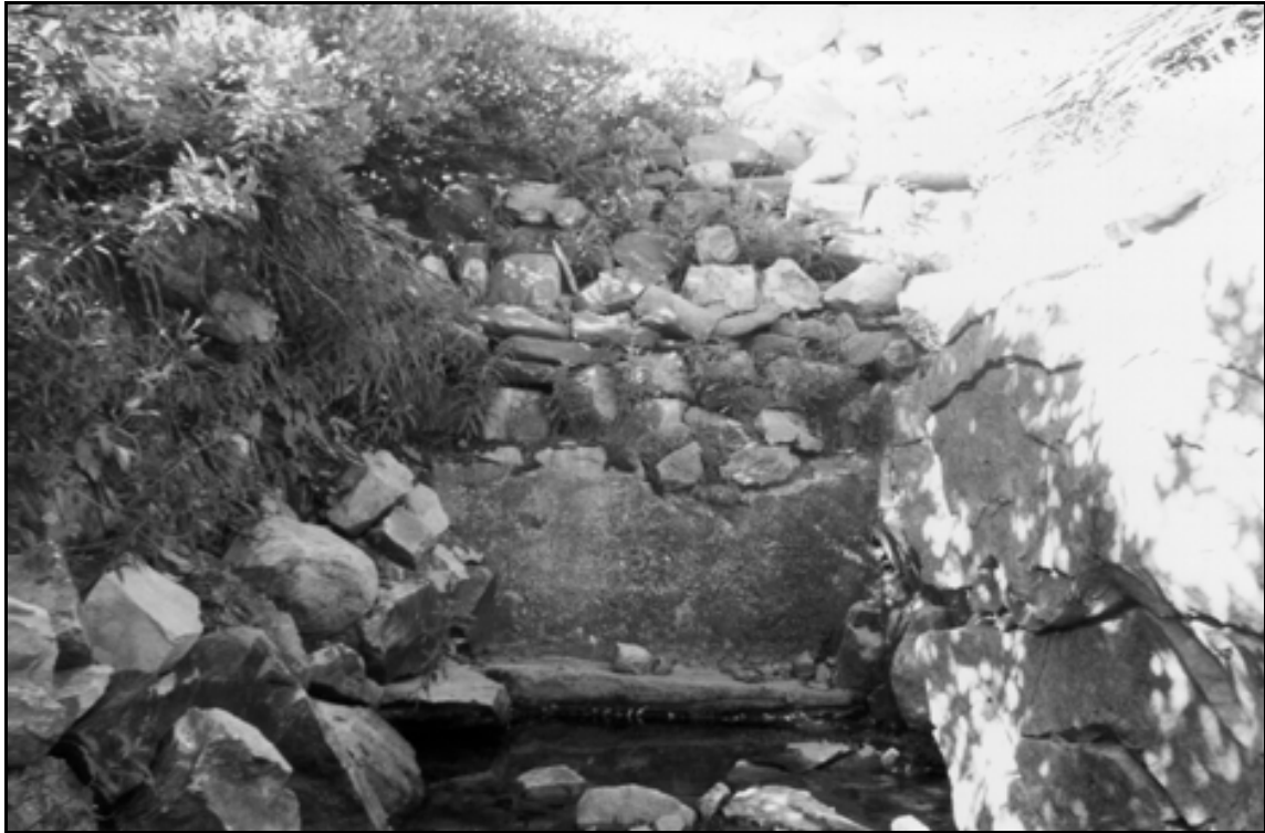
HAER UT-42-L. Superior Lake Dam. Overview of downstream outlet looking upstream; view to the north-northwest.
