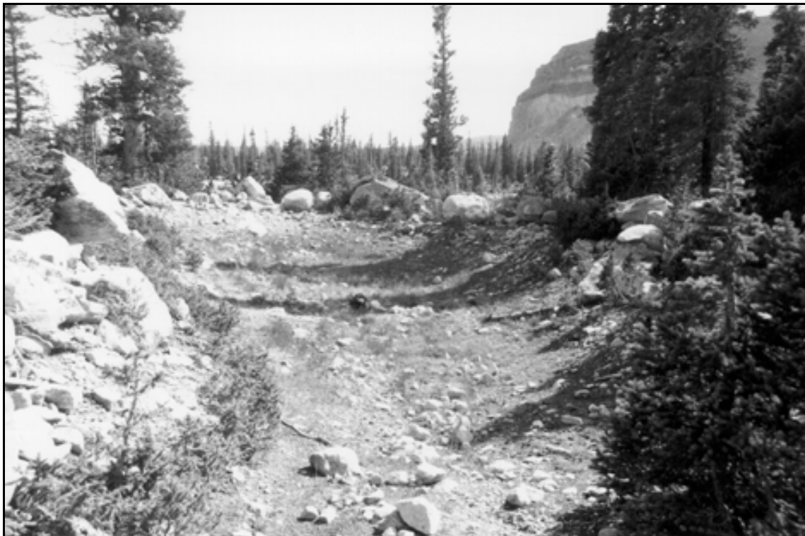
HAER UT-42-A. Bluebell Lake Dam. Overview of barrow area in south end of Dam #1; view to the south.
