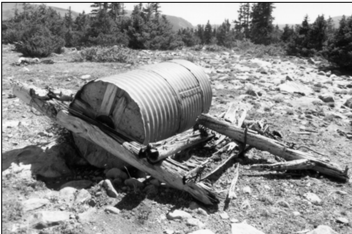
HAER UT-42-H. Five Point Lake Dam. Detail of stock-drawn earth roller with a log tongue; close-up view.
