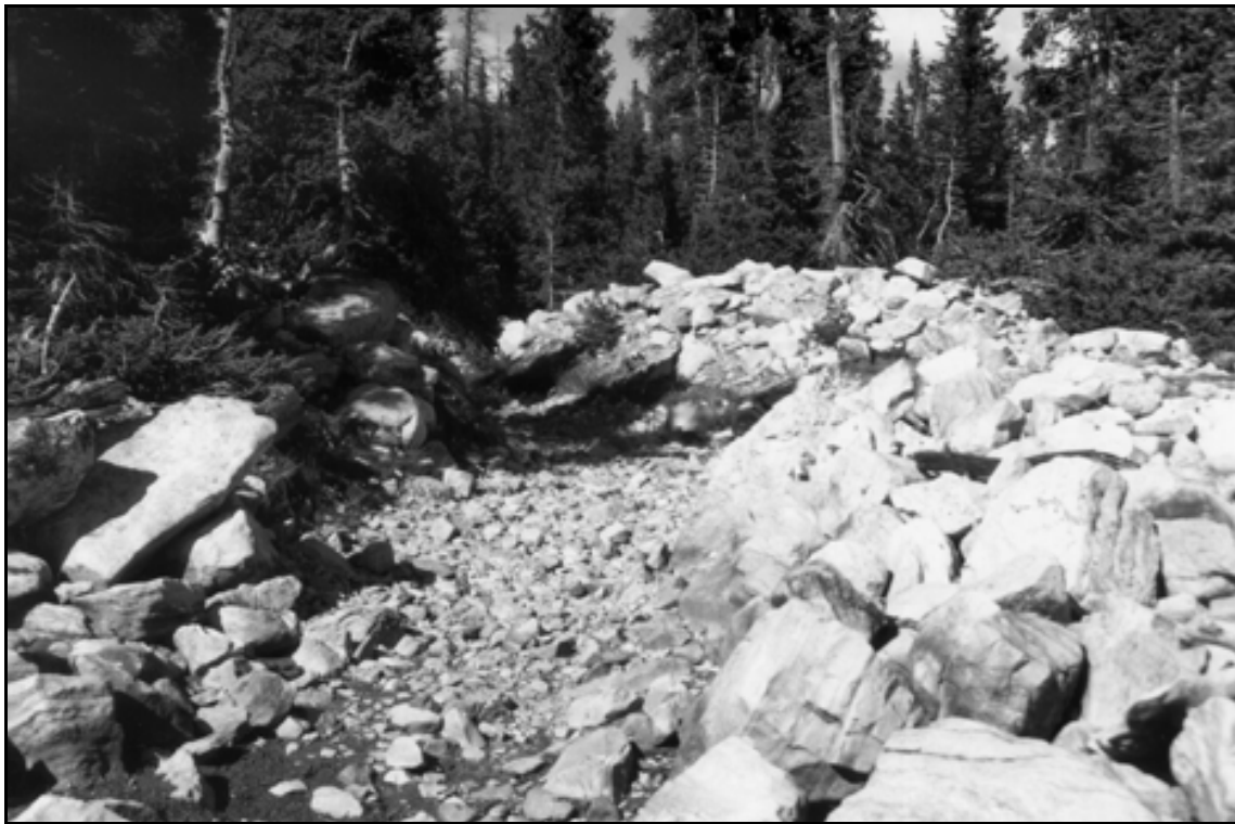
HAER UT-42-A. Bluebell Lake Dam. Overview of overflow spillway at Dam #1; view to the north-northeast.
