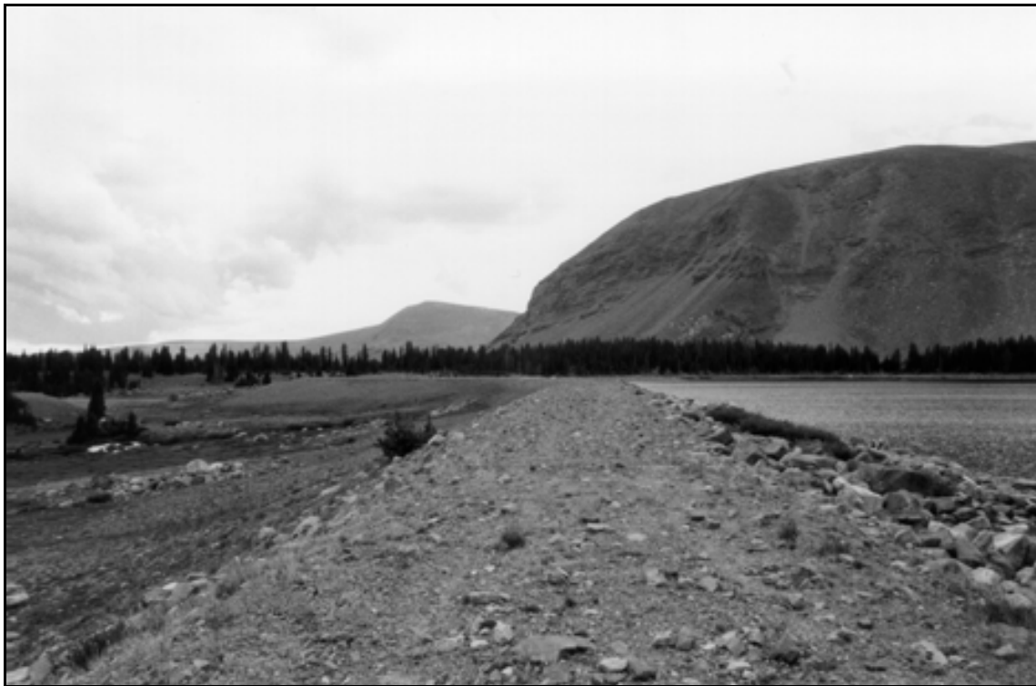
HAER UT-42-F. East Timothy Lake Dam. Dam overview from the east end; view to the west-southwest.
