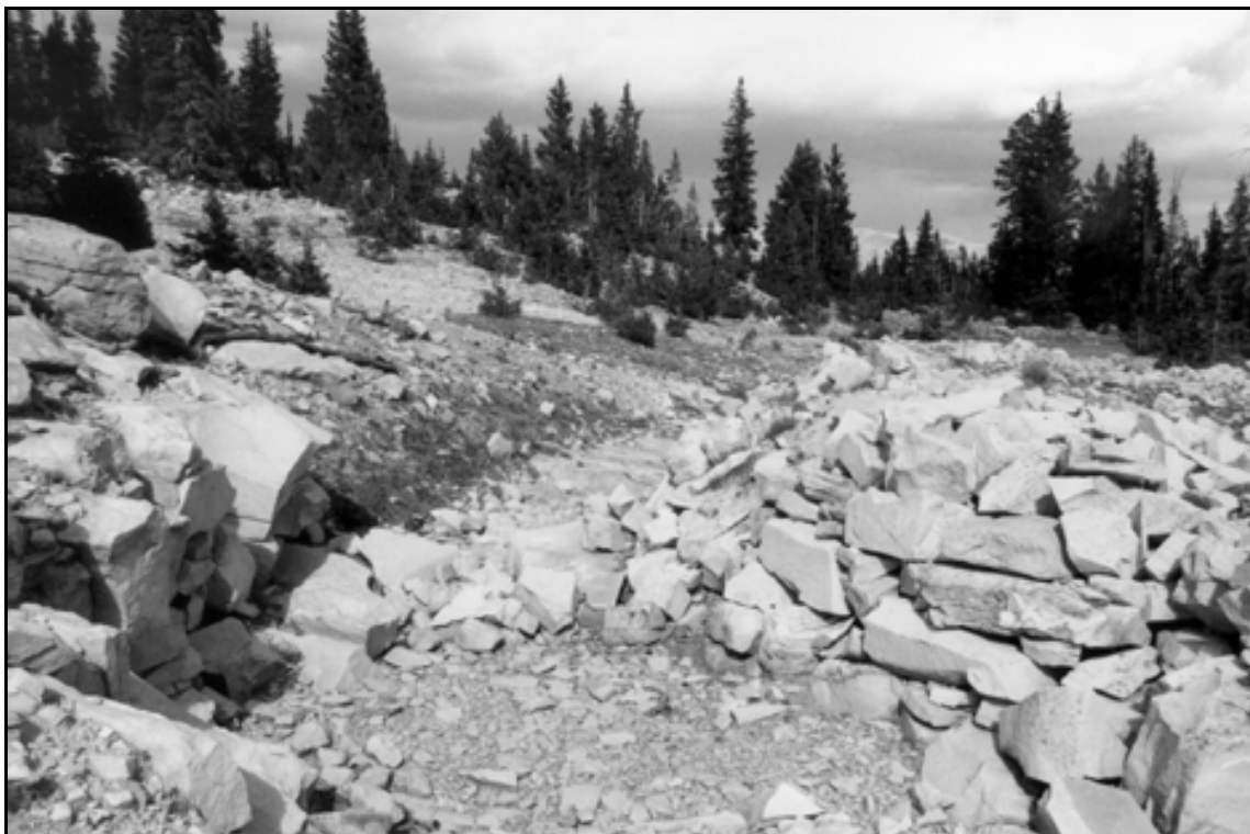
HAER UT-42-E. Drift Lake Dam. Overview of spillway at north end of dam; view to the northeast.
