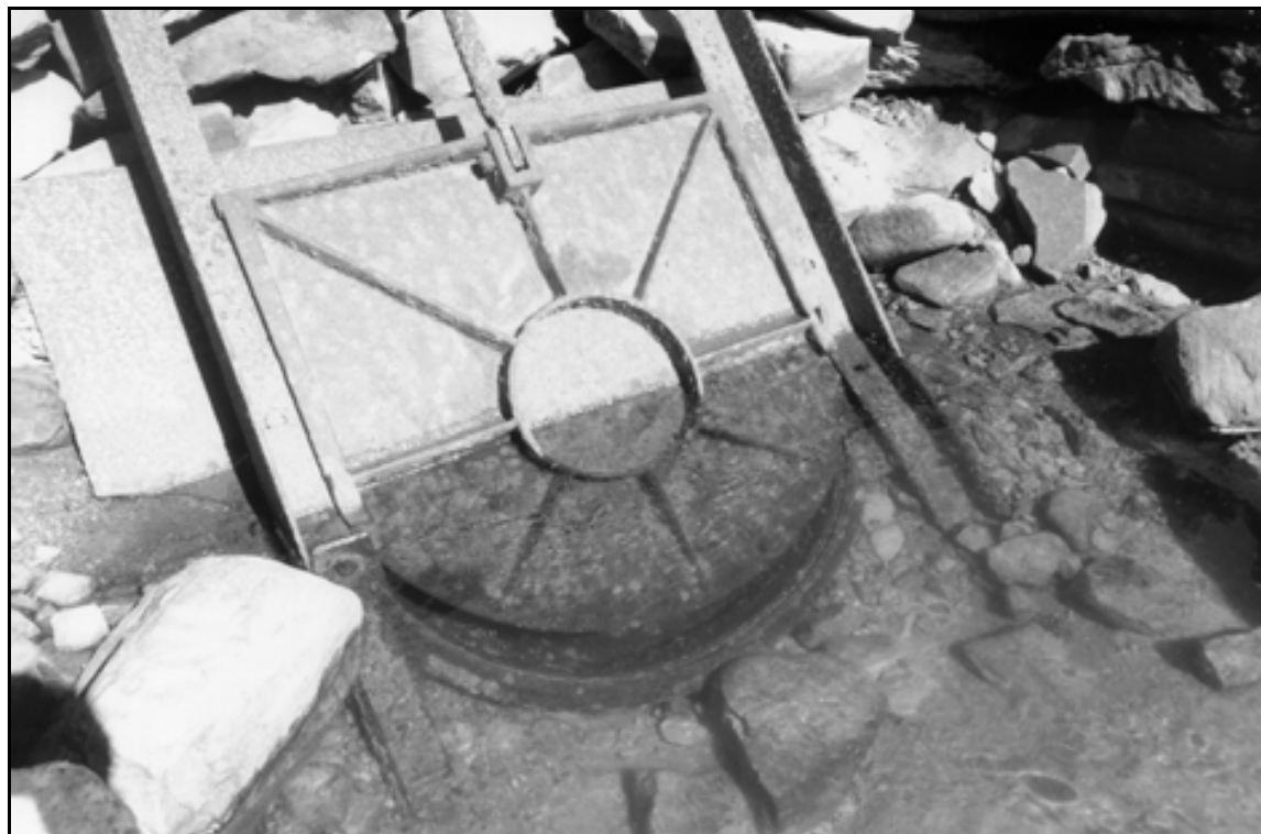
HAER UT-42-A. Bluebell Lake Dam. Headgate at Dam #1; close-up view.
