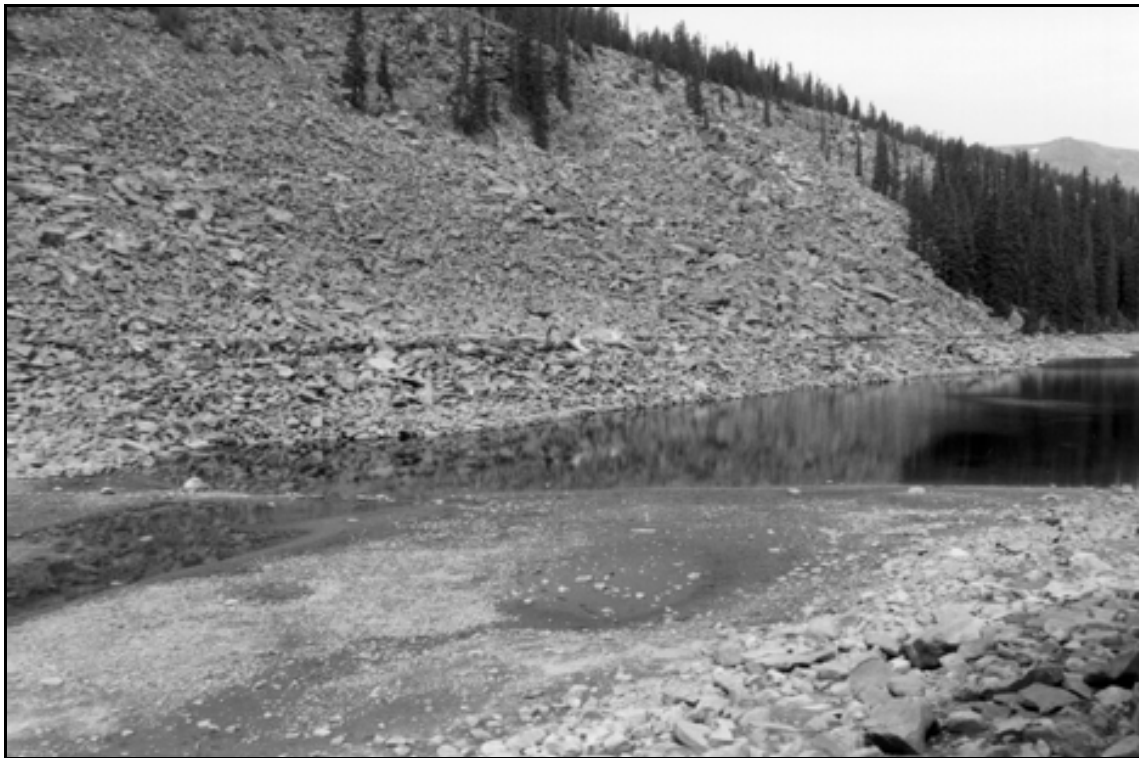
HAER UT-42-D. Deer Lake Dam. View of western shoreline during low water; view to the west.
