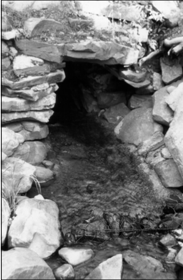
HAER UT-42-D. Deer Lake Dam. Downstream outlet looking toward the dam showing wire-reinforced concrete flooring and stone walls of outlet tunnel; view to the north.
