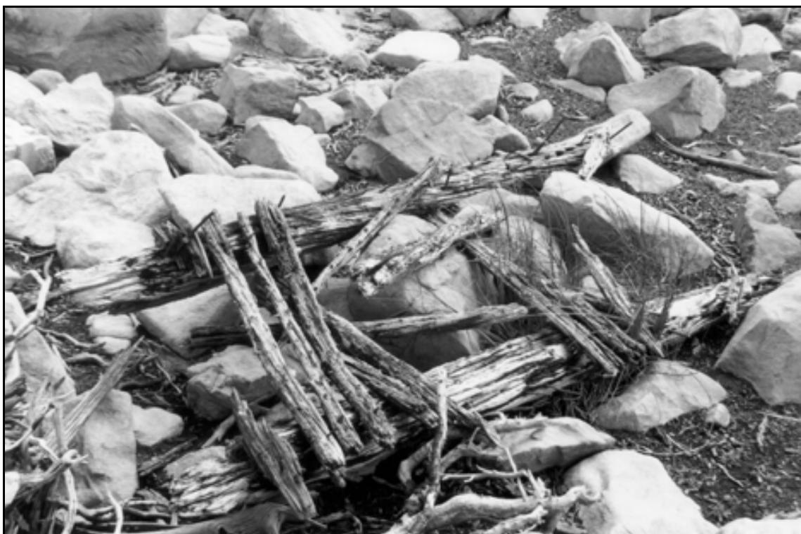
HAER UT-42-A. Bluebell Lake Dam. Detail of wooden framework with nails near south end of Dam #2; close-up view.
