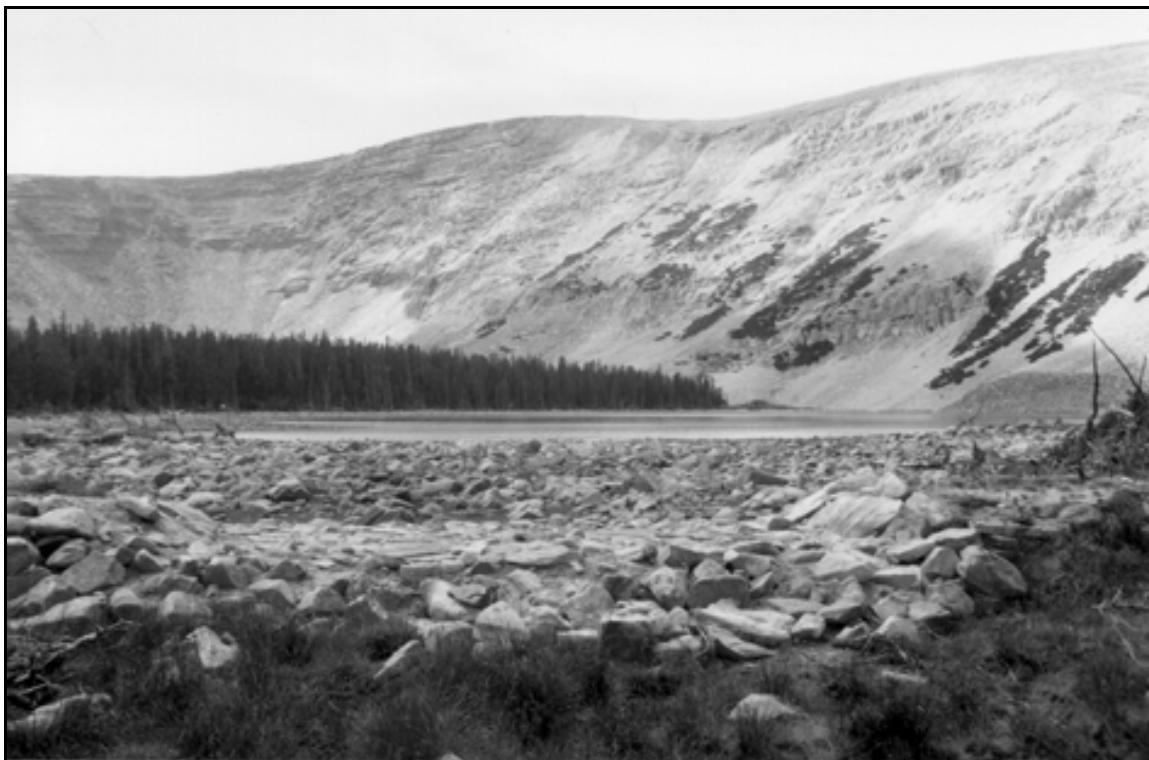
HAER UT-42-A. Bluebell Lake Dam. Overview of overflow spillway at Dam #2; view to the west-southwest.
