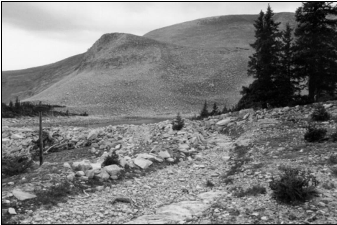
HAER UT-42-E. Drift Lake Dam. Overview of spillway channel; view to the south.
