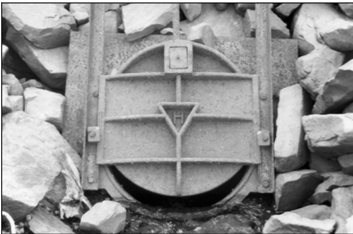
HAER UT-42-D. Deer Lake Dam. Headgate; close-up view.
