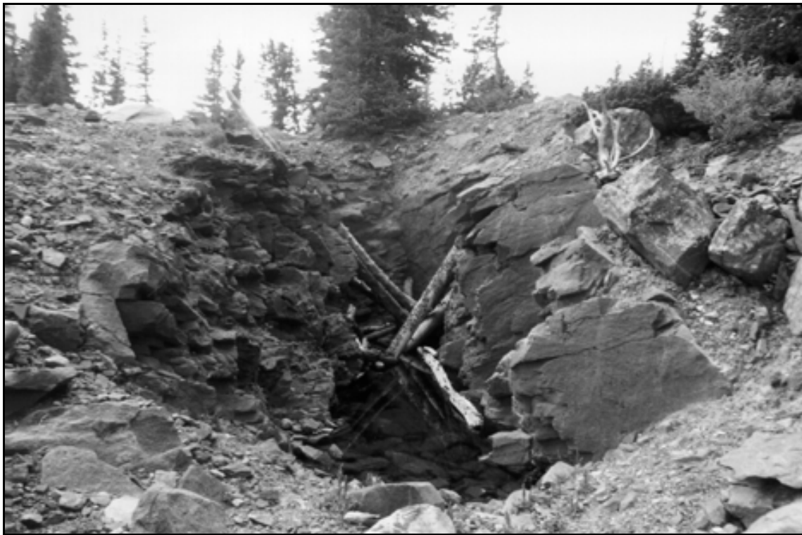
HAER UT-42-G. Farmers Lake Tunnel. View of tunnel inlet showing remains of log grizzly; view to the south.
