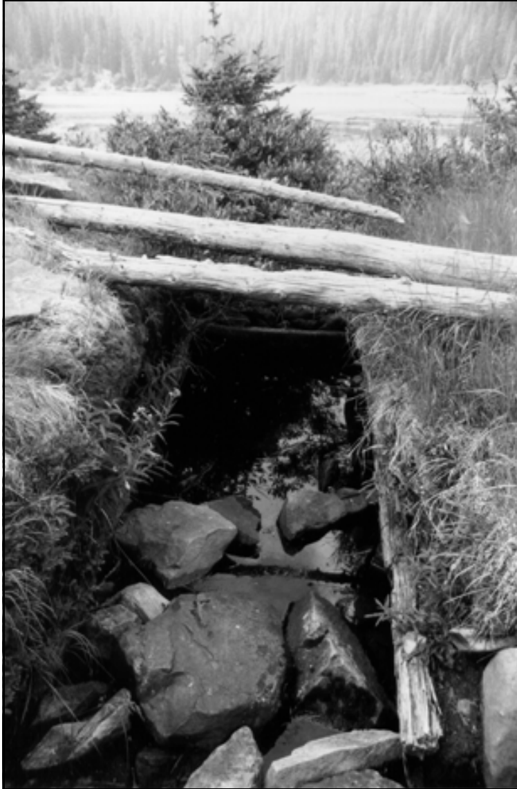
HAER UT-42-O. White Miller Lake Dam. Overview of wooden headgate & downstream outlet weir; view to the north.
