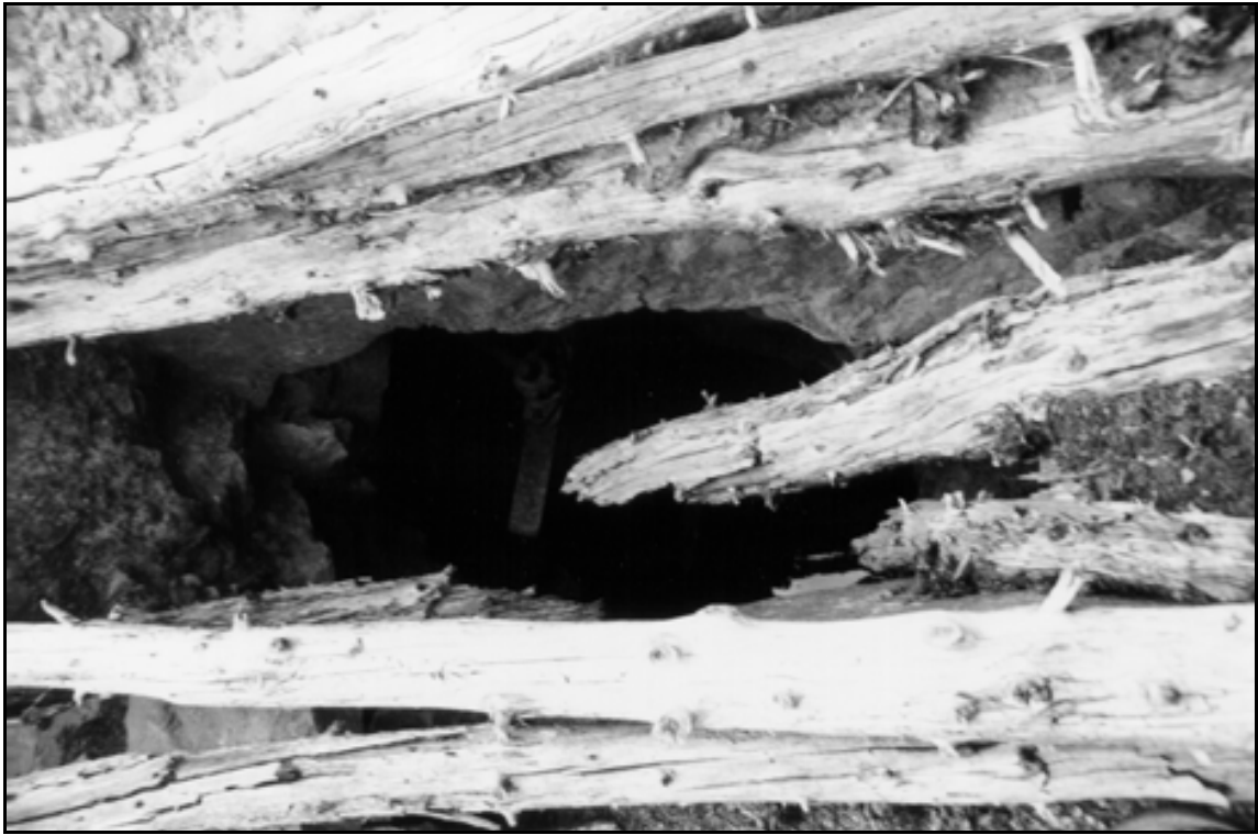
HAER UT-42-G. Farmers Lake Tunnel. View of cribbed gate control shaft looking down shaft at control device; close-up view.
