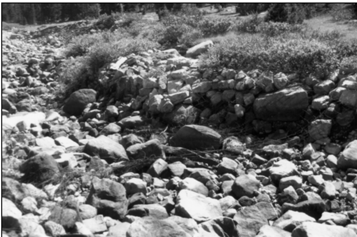
HAER UT-42-H. Five Point Lake Dam. Detail of reinforced area of spillway; view to the south-southeast.
