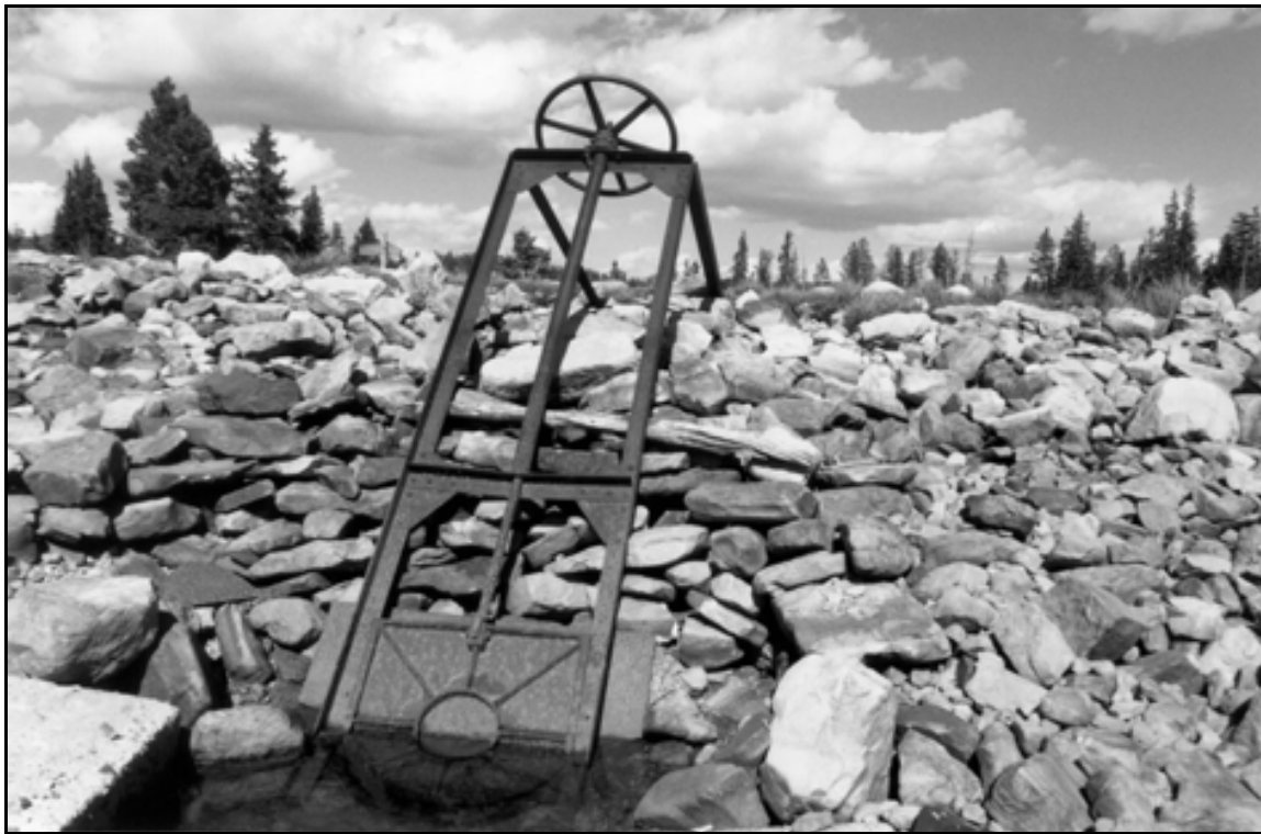
HAER UT-42-A. Bluebell Lake Dam. Overview of gate lift mechanism on upstream outlet at Dam #1; view to the northeast.
