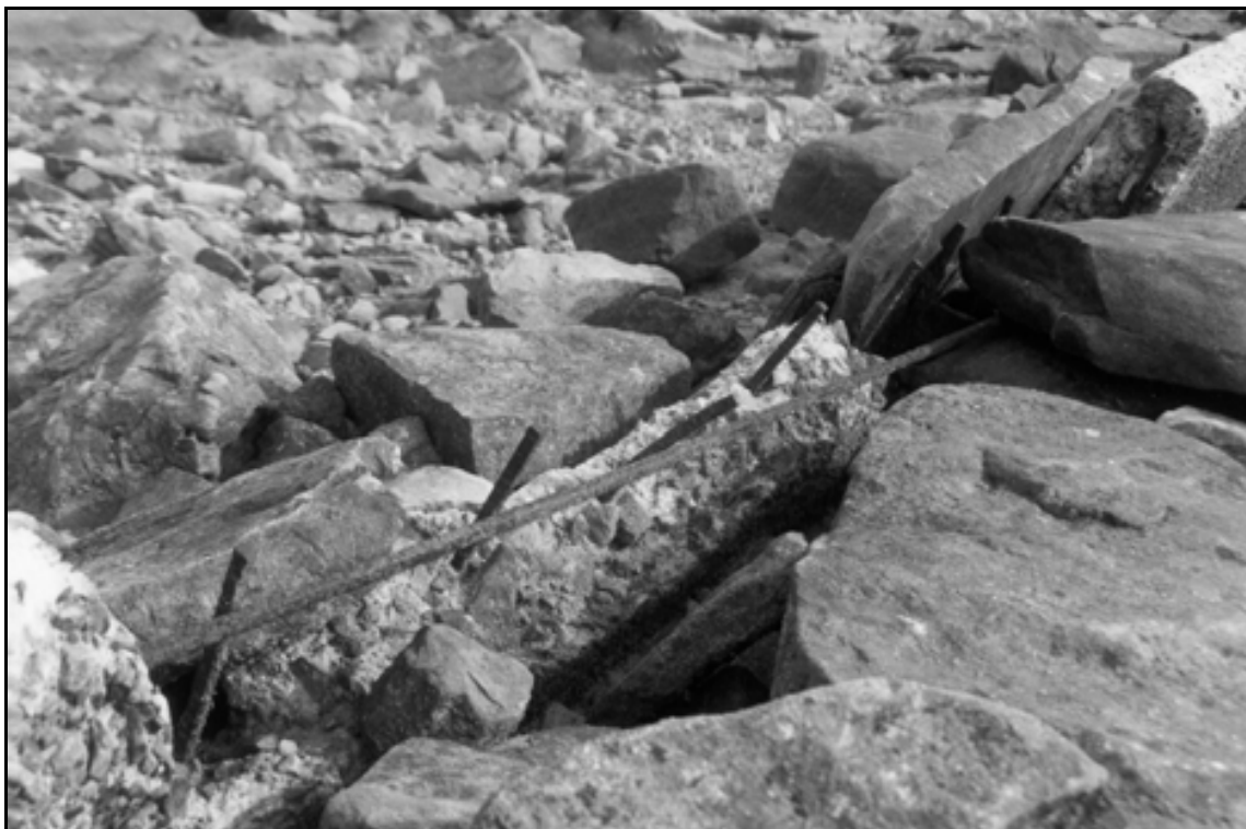
HAER UT-42-H. Five Point Lake Dam. Rebar reinforcement exposed in damaged section of curb along overflow spillway; close-up view.
