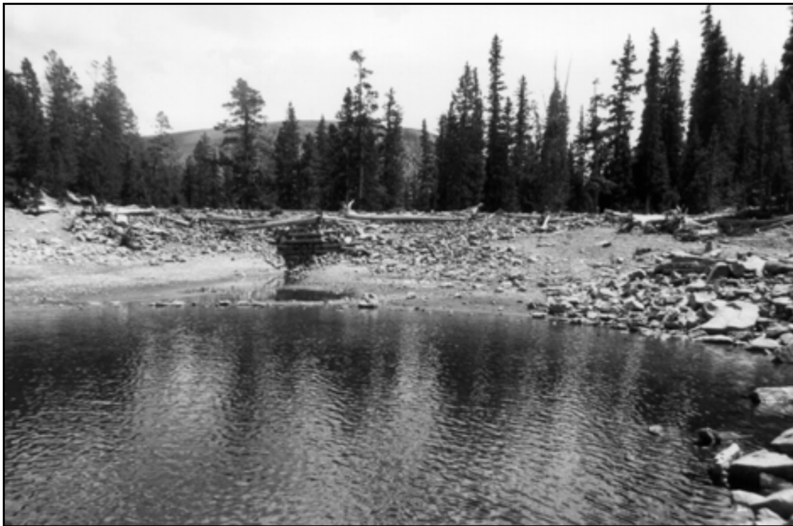
HAER UT-42-D. Deer Lake Dam. Overview showing profile of dam from the low water mark; view to the southeast.
