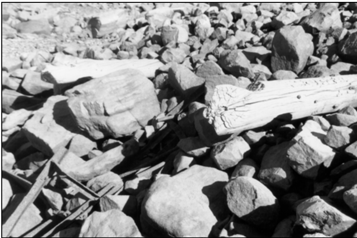
HAER UT-42-L. Superior Lake Dam. Remnants of previous log cribbing structure before dam was modified; close-up view to the east.
