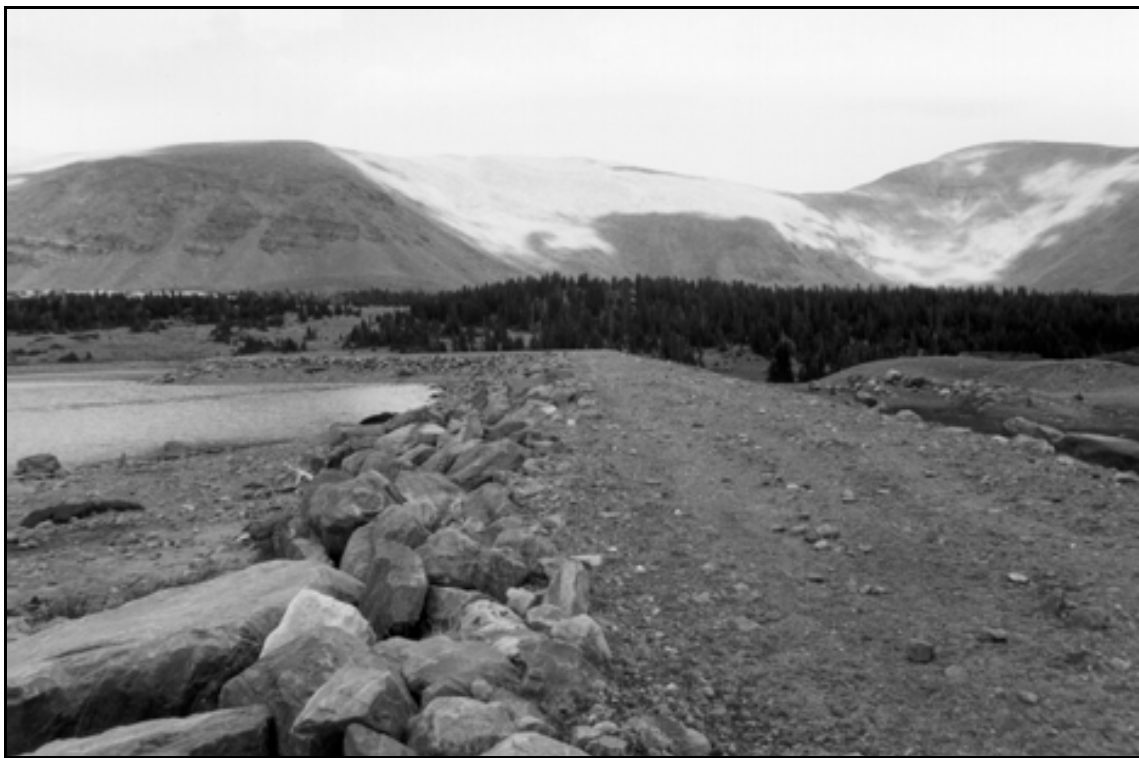
HAER UT-42-F. East Timothy Lake Dam. Dam overview from the west end; view to the northeast.
