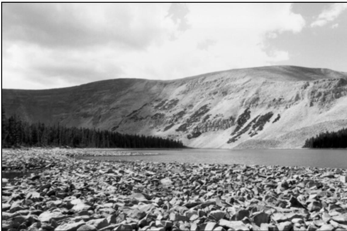
HAER UT-42-A. Bluebell Lake Dam. Overview of lake; view to the south.
