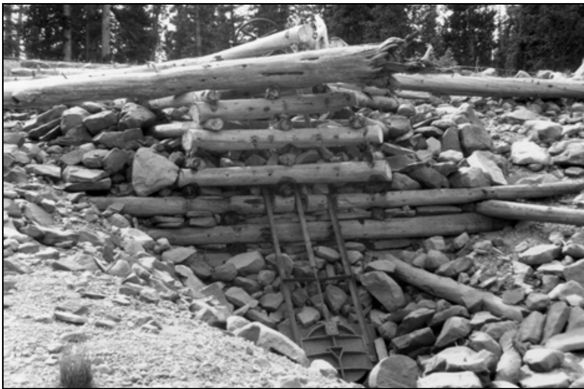
HAER UT-42-D. Deer Lake Dam. Overview of headgate, cribbing, and platform on upstream face of dam; view to the south.
