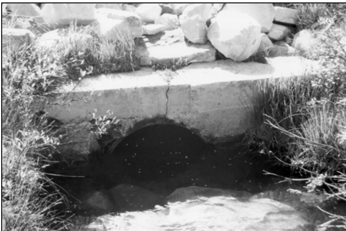
HAER UT-42-A. Bluebell Lake Dam. Overview of downstream outlet at Dam #1; close-up view.
