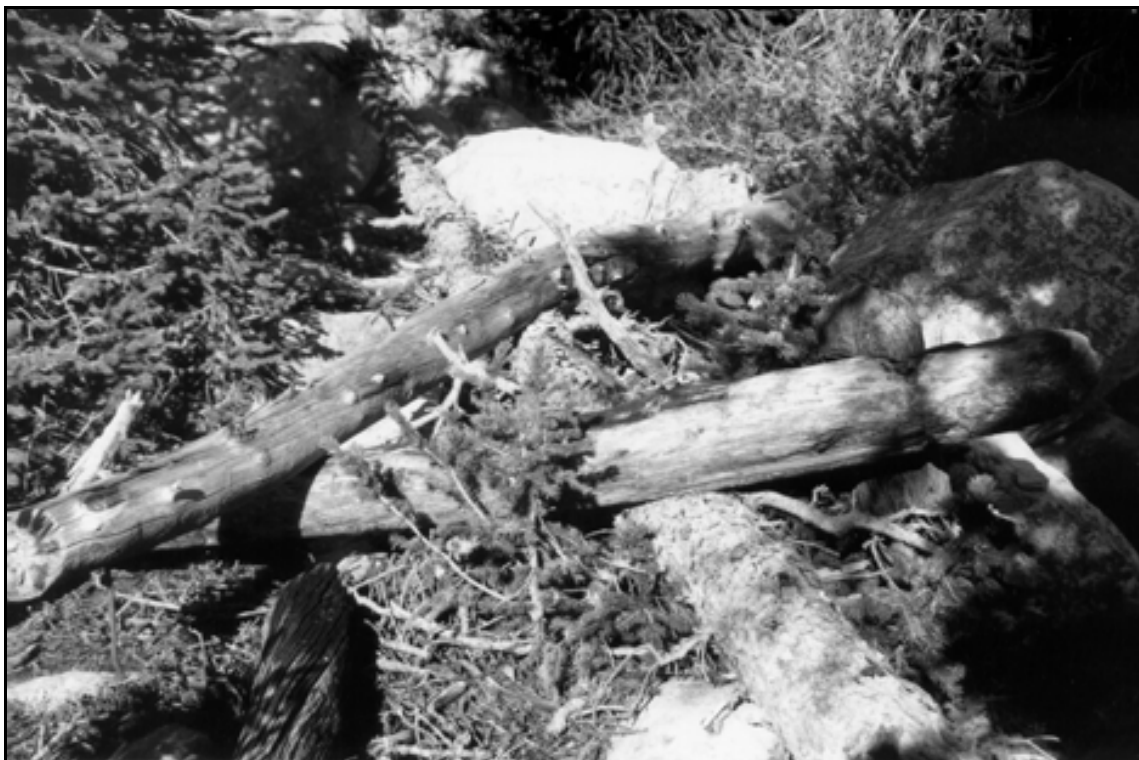
HAER UT-42-A. Bluebell Lake Dam. Notched log remnants in spillway at Dam #1; close-up view.
