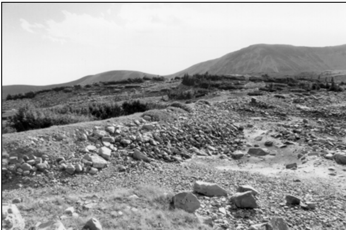
HAER UT-42-L. Superior Lake Dam. Overview of upstream face of dam; view to the southwest.
