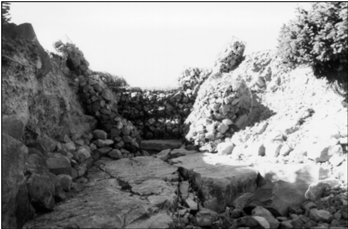
HAER UT-42-L. Superior Lake Dam. Overview of lower level of spillway looking upstream toward upper level; view to the northwest.
