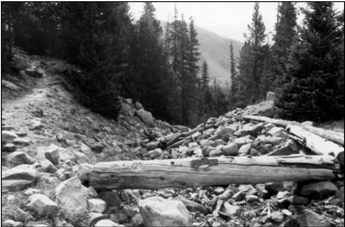
HAER UT-42-D. Deer Lake Dam. Overview looking downstream at overflow spillway from the north end of the dam. Swift Creek Trail is visible in left side of frame and remnants of possible footbridge in foreground; view to the southeast.
