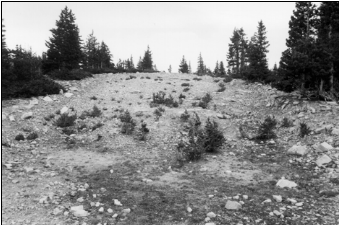
HAER UT-42-E. Drift Lake Dam. Overview of barrow area at south end of dam; view to the southeast.
