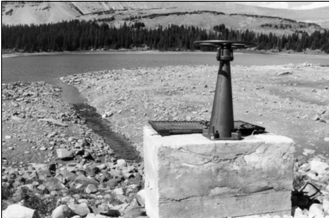
HAER UT-42-H. Five Point Lake Dam. Overview of dam control box, upstream outlet channel and lake in background; view to the west-northwest.
