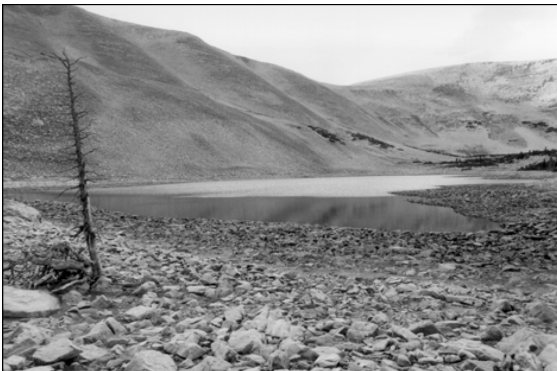
HAER UT-42-E. Drift Lake Dam. Overview of lake from south end of dam; view to the northwest.
