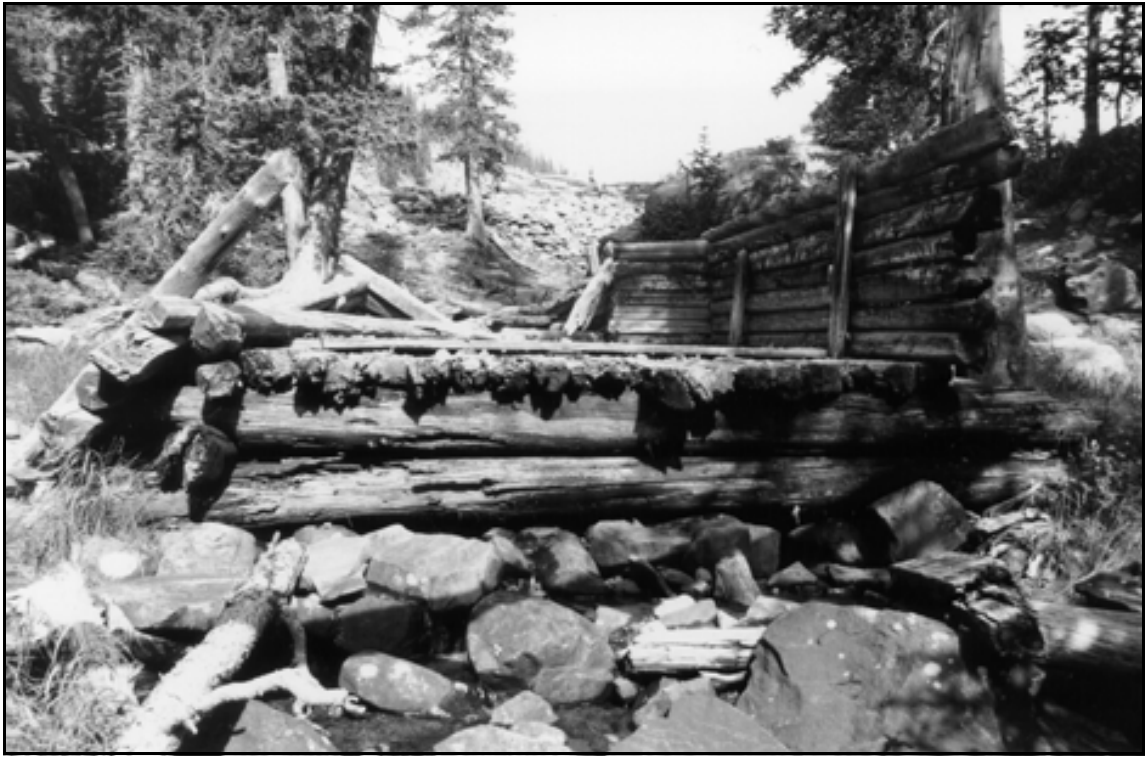
HAER UT-42-D. Deer Lake Dam. Overview of possible measuring weir downstream from dam; view looking upstream to the northwest.
