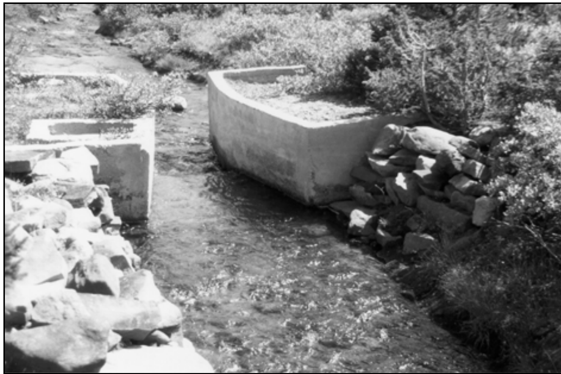
HAER UT-42-H. Five Point Lake Dam. Overview of check dam/gauging box and downstream outlet channel; view to the east-southeast.
