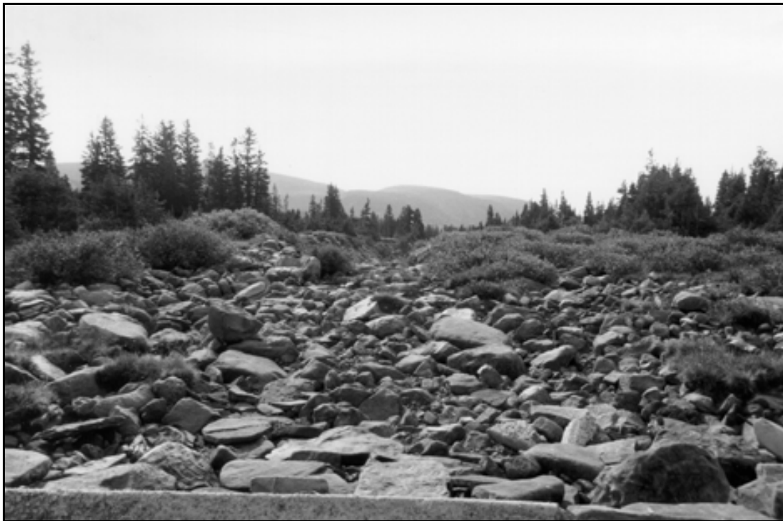
HAER UT-42-H. Five Point Lake Dam. Overview of overflow spillway downstream channel from concrete curb; view to the southeast.
