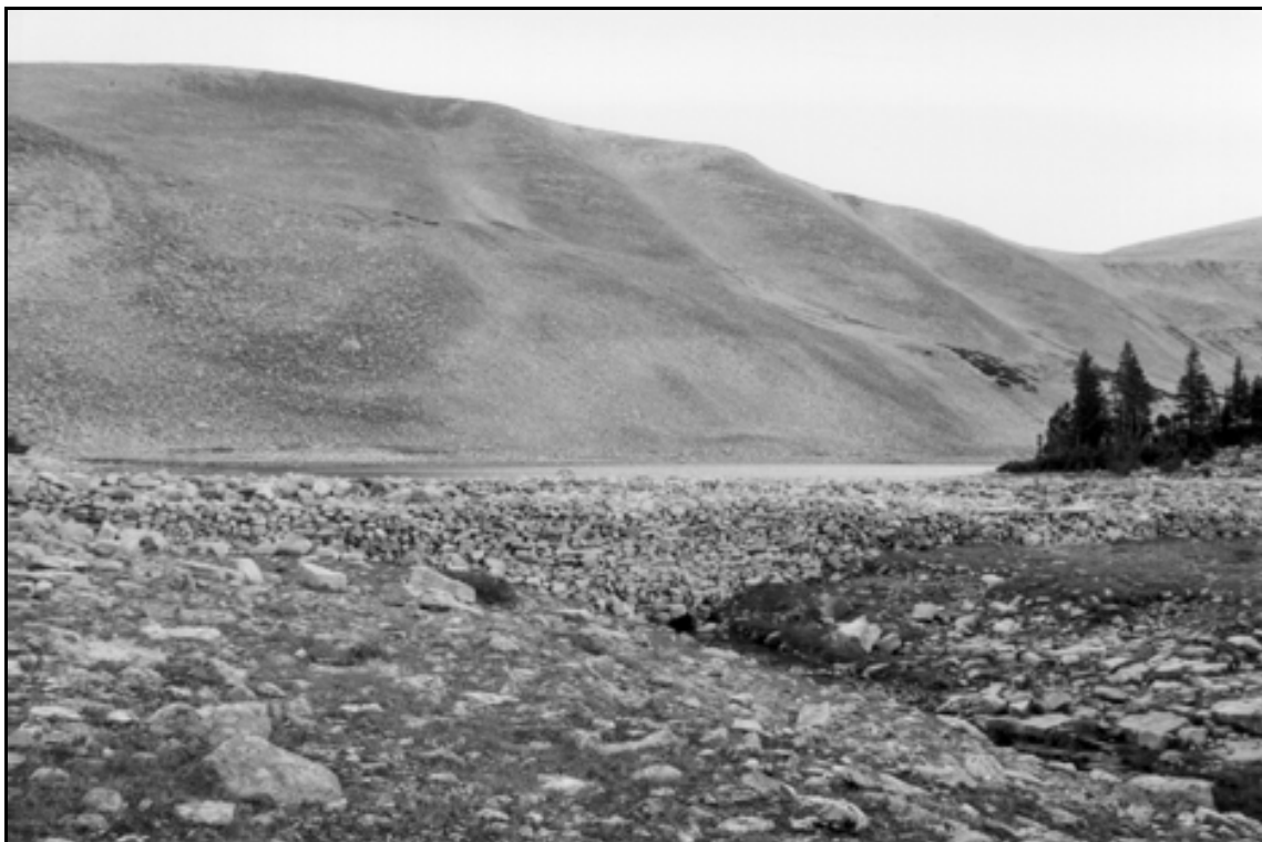
HAER UT-42-E. Drift Lake Dam. Overview of downstream outlet and east side of dam; view to the northwest.
