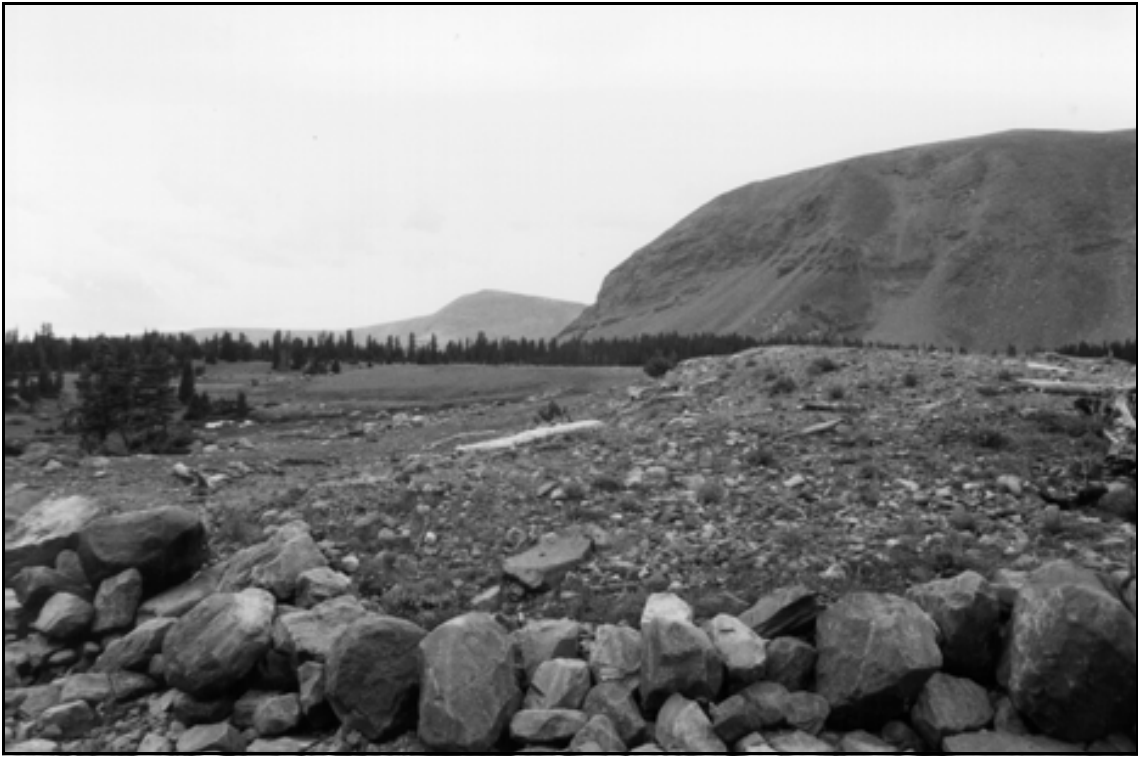
HAER UT-42-F. East Timothy Lake Dam. Dam overview with spillway in foreground; view to the southwest.
