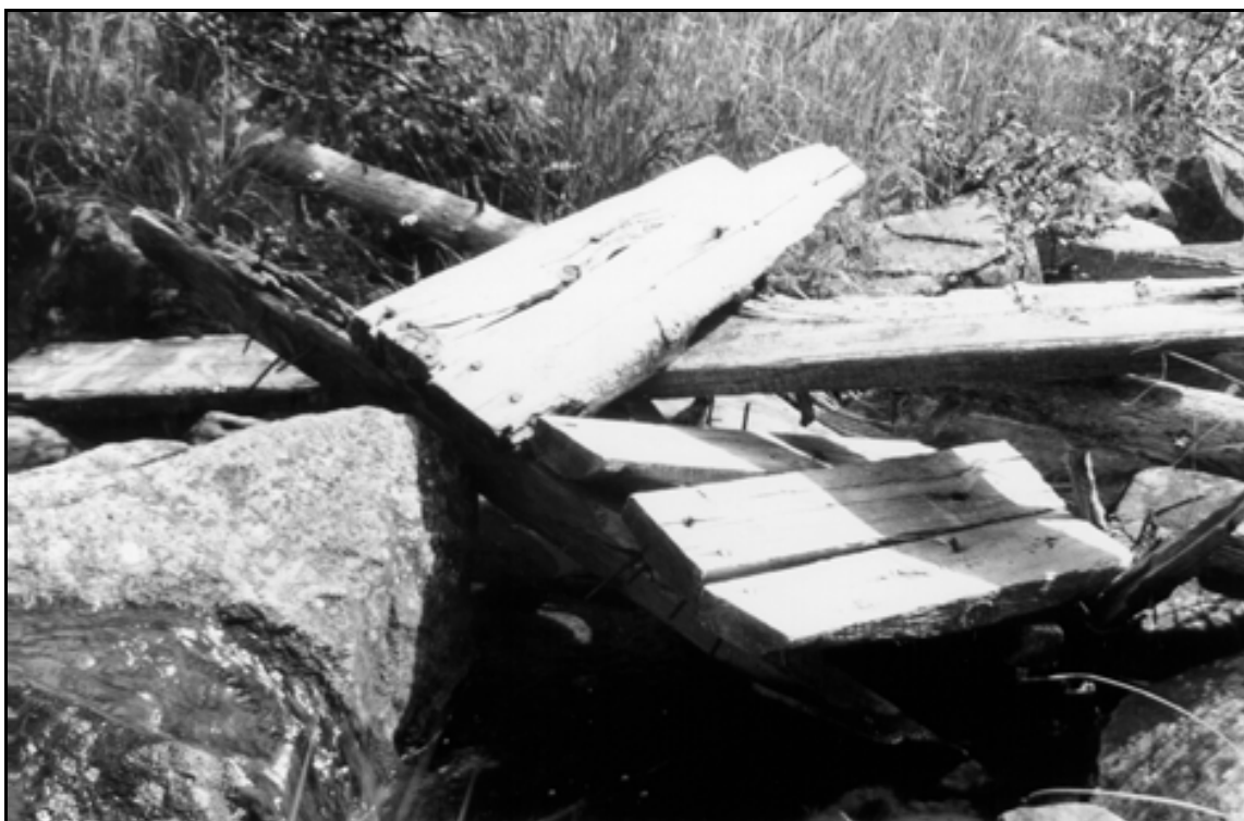
HAER UT-42-D. Deer Lake Dam. Collapsed wooden footbridge across downstream outlet channel; close-up view to the east.
