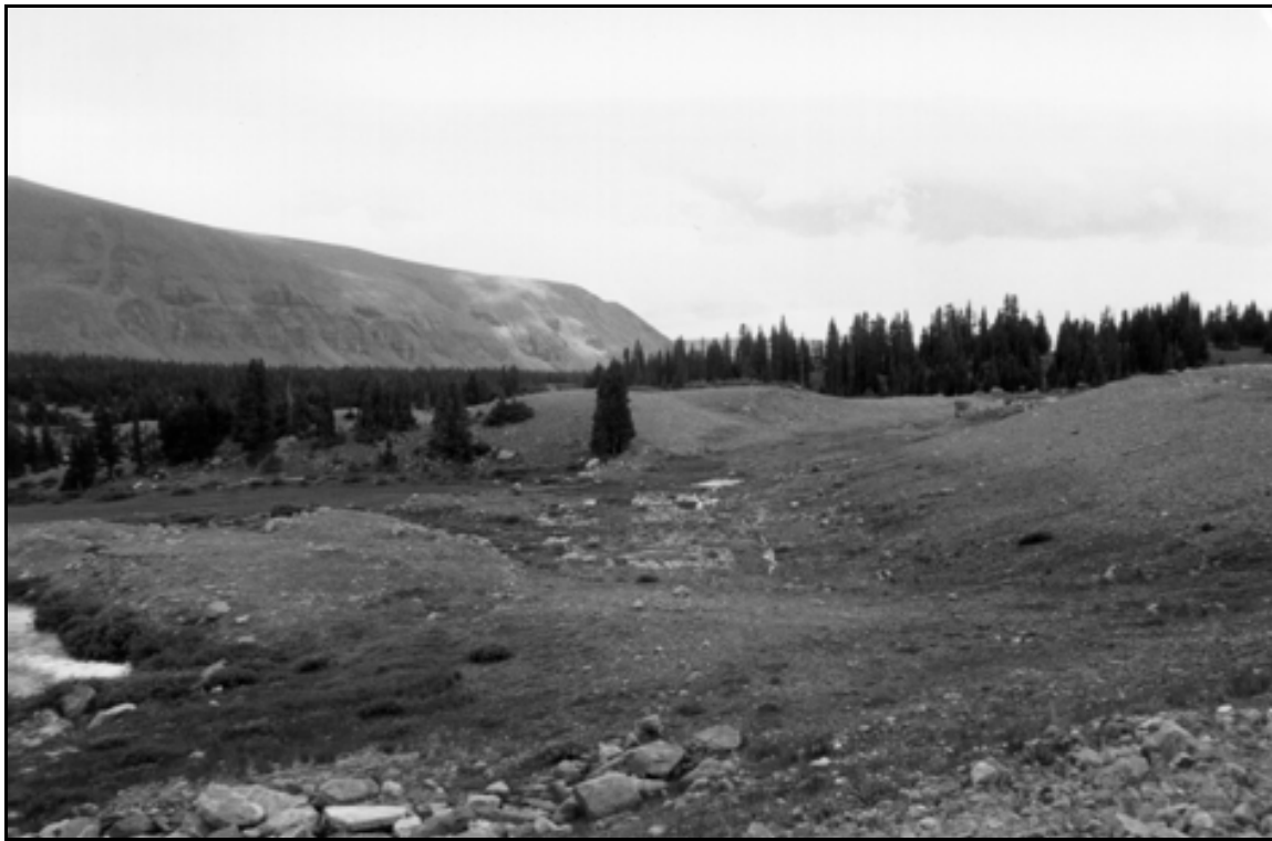
HAER UT-42-F. East Timothy Lake Dam. Overview from the dam across the outlet channel; view to the south.
