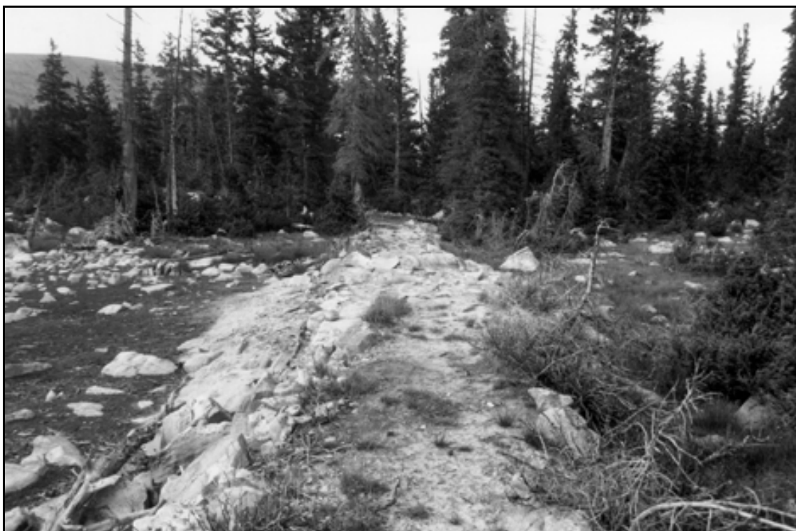
HAER UT-42-A. Bluebell Lake Dam. Overview of dam surface at north end of Dam #2; view to the north-northwest.
