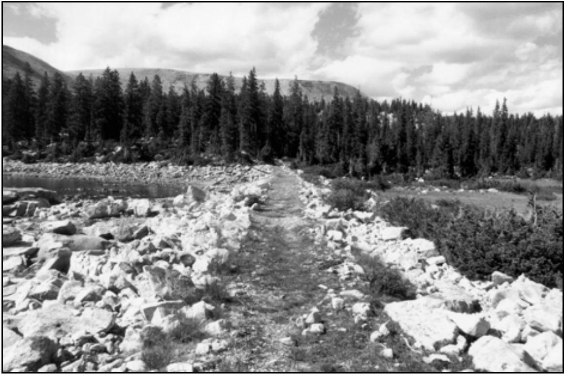
HAER UT-42-A. Bluebell Lake Dam. Overview of dam surface at Dam #1; view to the northwest.
