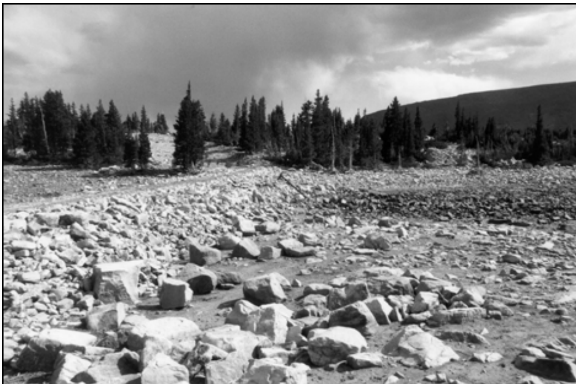
HAER UT-42-E. Drift Lake Dam. Overview of west face of dam; view to the southeast.
