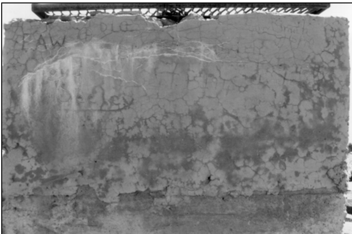
HAER UT-42-H. Five Point Lake Dam. Detail of west face of control box showing inscriptions; close-up view.
