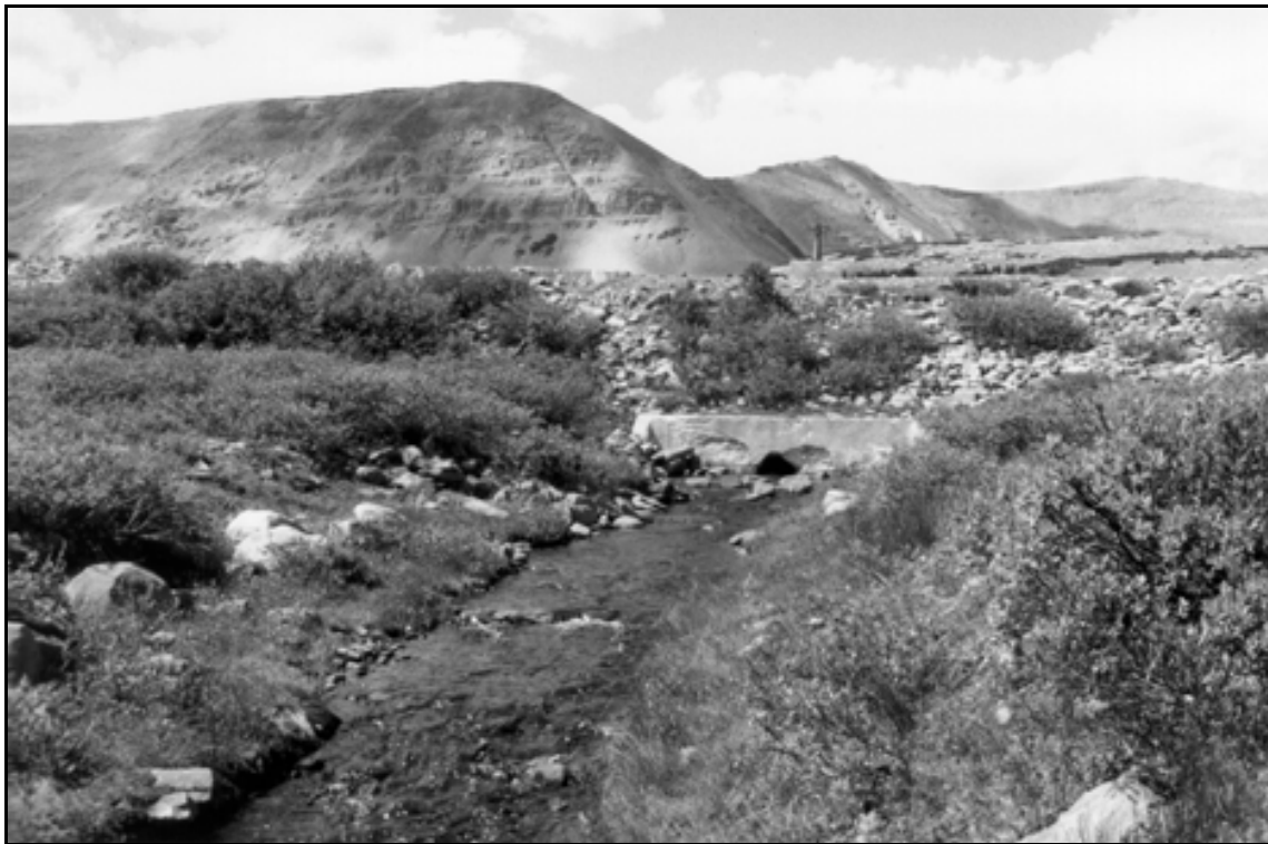
HAER UT-42-H. Five Point Lake Dam. Overview of downstream outlet, control box, and east face of dam; view to the west.
