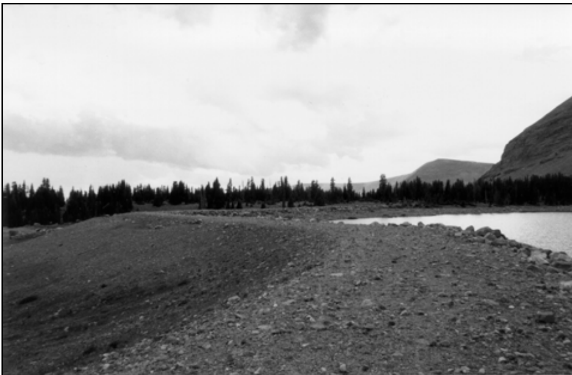
HAER UT-42-F. East Timothy Lake Dam. Overview of the southwest portion of the dam looking across culvert; view to the southwest.
