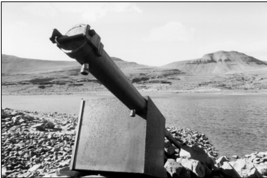
HAER UT-42-L. Superior Lake Dam. Control box showing Superior Lake in background; close-up view to the west.
