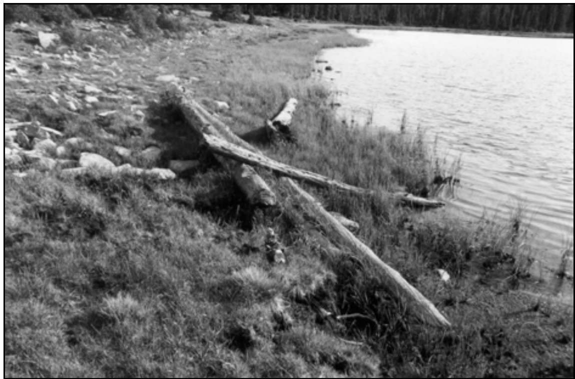
HAER UT-42-O. White Miller Lake Dam. Overview of lake with unidentified wooden structure in foreground; view to the south-southwest.
