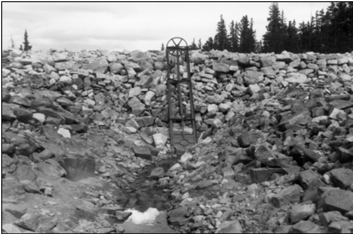
HAER UT-42-E. Drift Lake Dam. Overview of gate lift mechanism and handwheel; view to the east-northeast.
