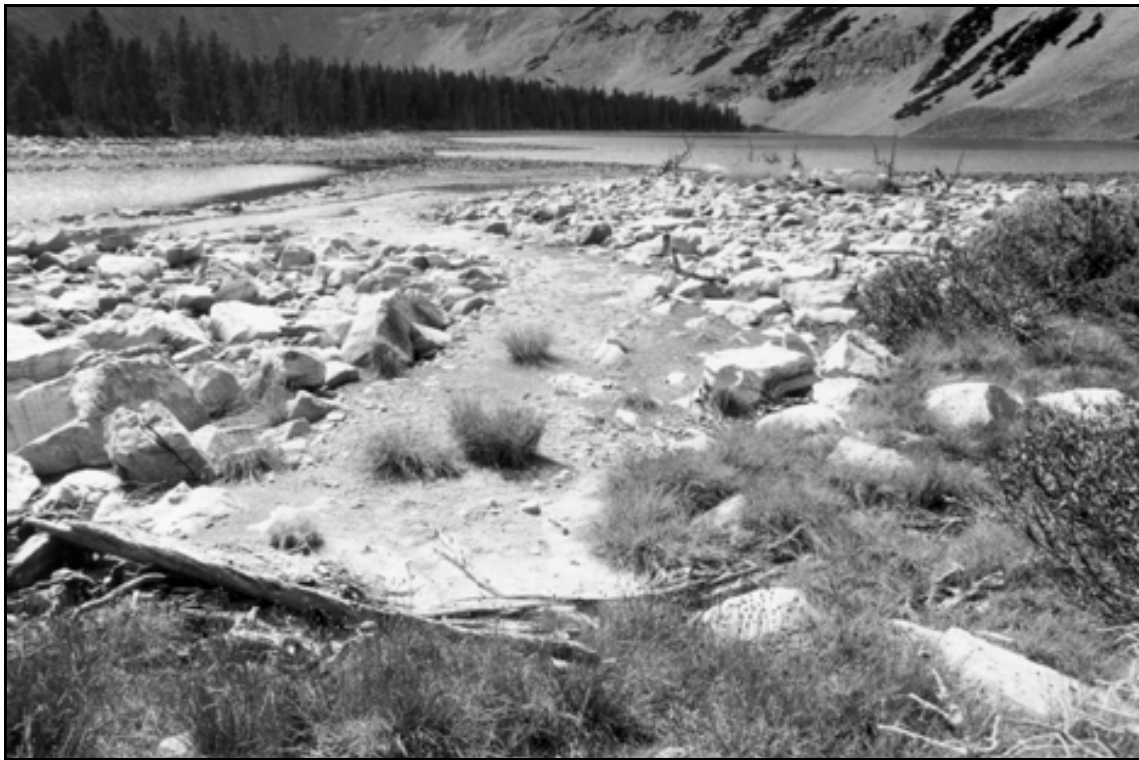
HAER UT-42-A. Bluebell Lake Dam. Overview of dam Ramp #1 from barrow area to Dam #2; view to the west-southwest.
