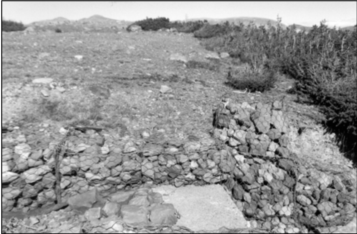
HAER UT-42-L. Superior Lake Dam. Northeast profile of spillway, showing wire cribbing detail and concrete step of upper level; view to the east-northeast.
