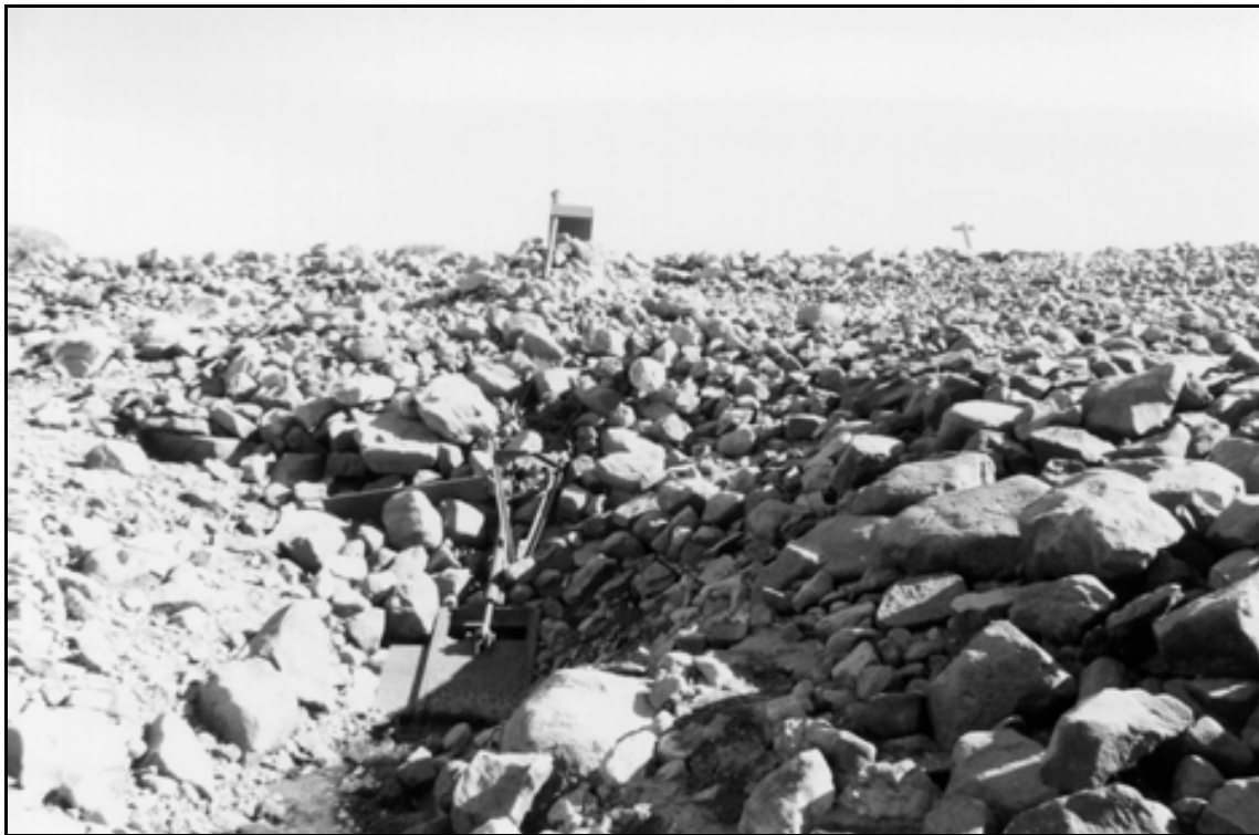
HAER UT-42-L. Superior Lake Dam. Overview of upstream face of dam showing headgate, control box, and top of dam; view to the southeast.
