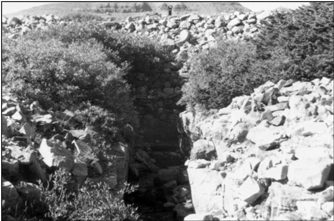
HAER UT-42-L. Superior Lake Dam. Overview of downstream outlet and channel looking upstream with top of dam in background; view to the north-northwest.
