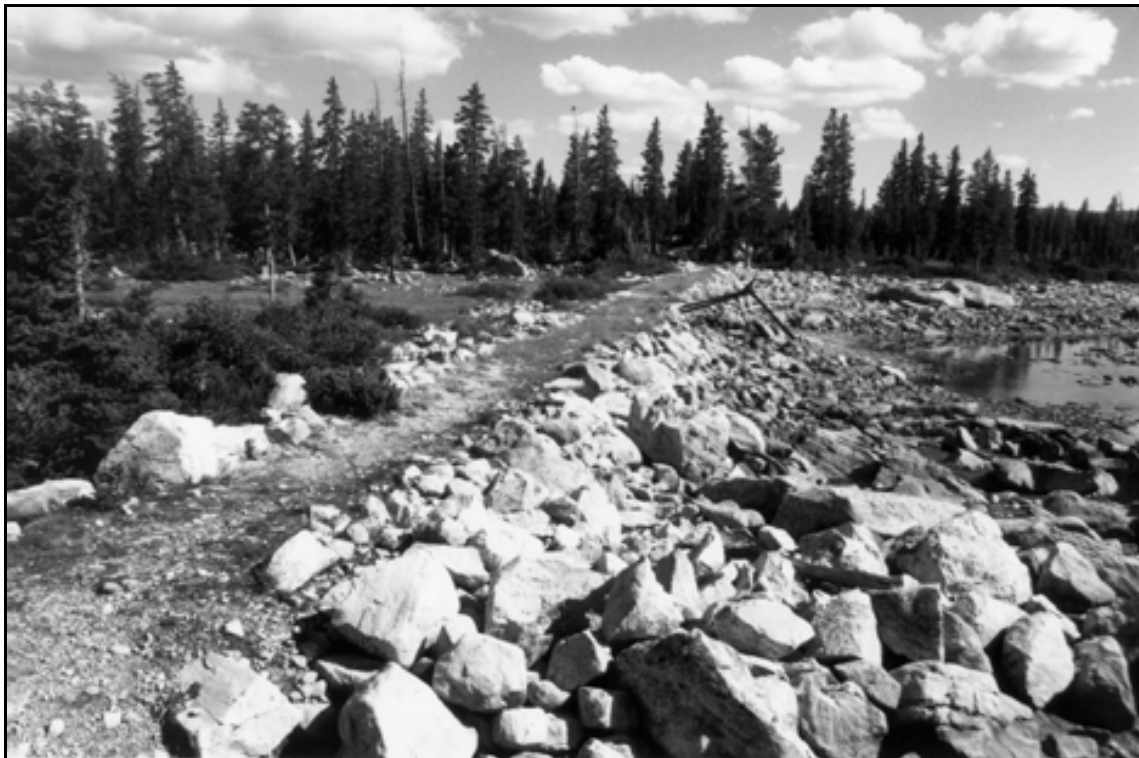
HAER UT-42-A. Bluebell Lake Dam. Overview of Dam #1; view to the south-southeast.
