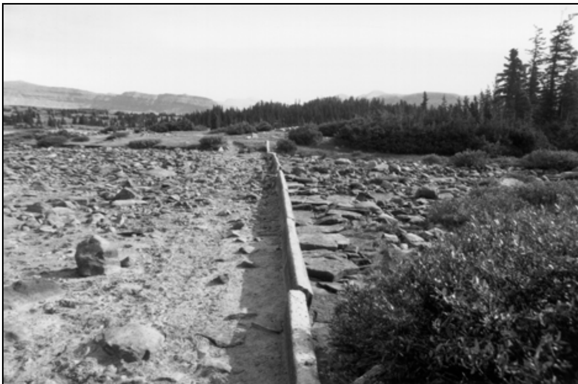
HAER UT-42-H. Five Point Lake Dam. Overview of overflow spillway concrete curb; view to the north-northeast.
