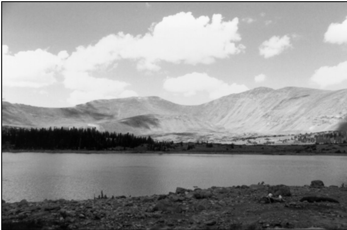
HAER UT-42-F. East Timothy Lake Dam. Lake overview; view to the north.
