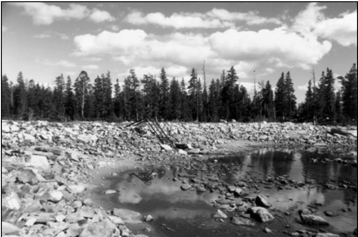
HAER UT-42-A. Bluebell Lake Dam. Overview of Dam #1 upstream outlet and west side of dam; view to the southeast.
