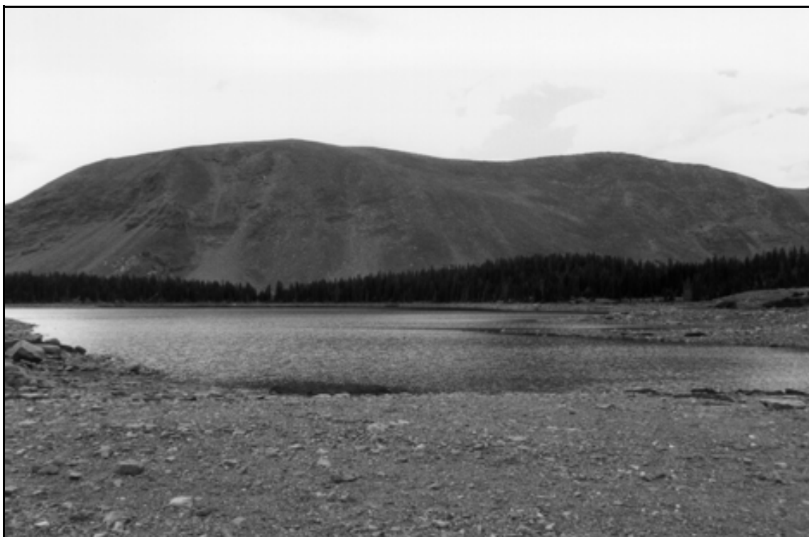
HAER UT-42-F. East Timothy Lake Dam. Lake overview from spillway; view to the west.
