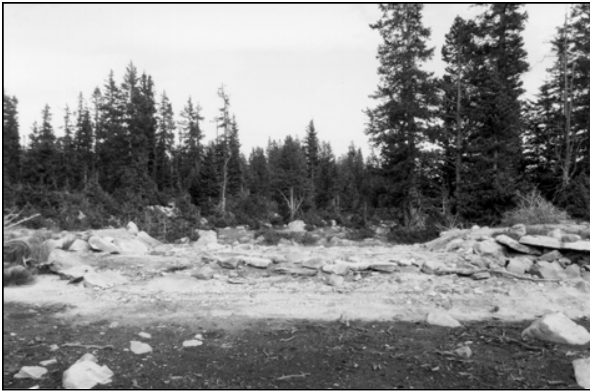
HAER UT-42-A. Bluebell Lake Dam. Overview of overflow spillway at Dam #2; view to the east-northeast.
