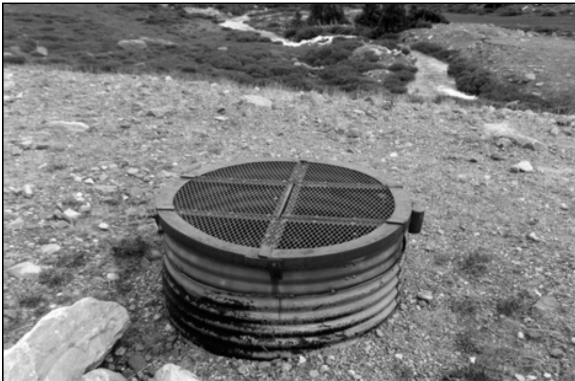
HAER UT-42-F. East Timothy Lake Dam. Overview of top of dam showing culvert shaft with outlet channel in background; view to the southeast.
