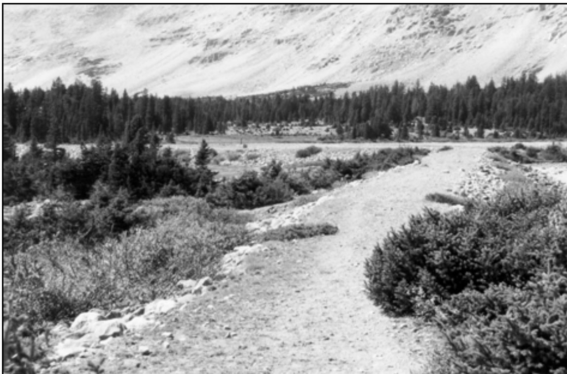
HAER UT-42-H. Five Point Lake Dam. Dam overview; view to the southwest.
