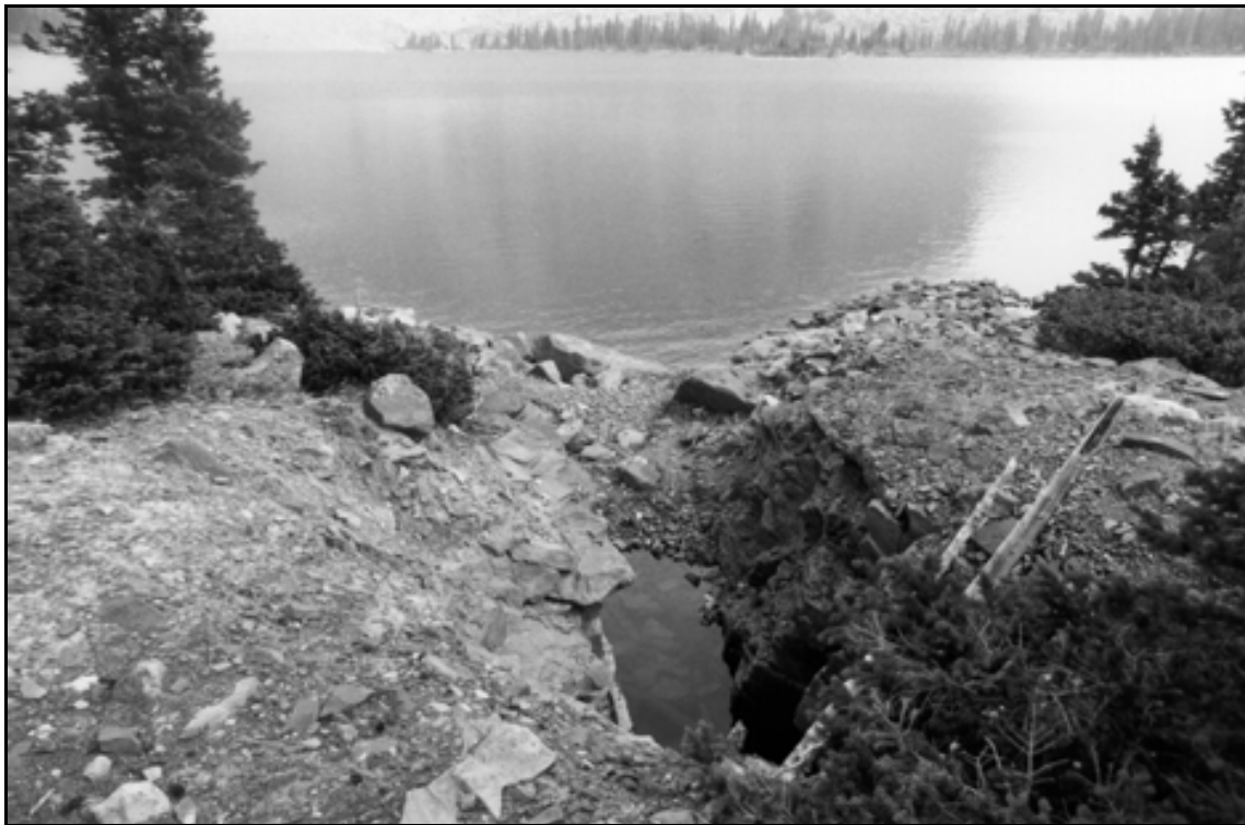
HAER UT-42-G. Farmers Lake Tunnel. View from atop the tunnel inlet showing upstream outlet channel and lake overview; view to the north.
