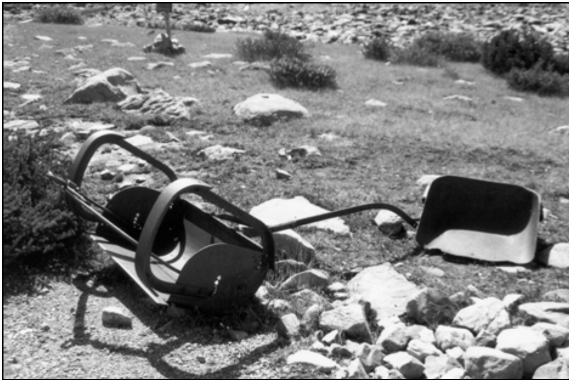
HAER UT-42-H. Five Point Lake Dam. Overview of stock-drawn earth scraper and stock-drawn shovel; close-up view.
