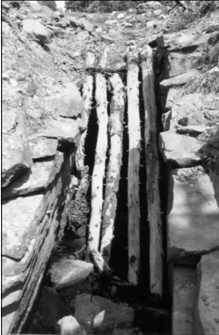
HAER 42-UT-G. Farmers Lake Tunnel. Overview of wooden grate trash rack and downstream outlet of tunnel; view to the northwest.
