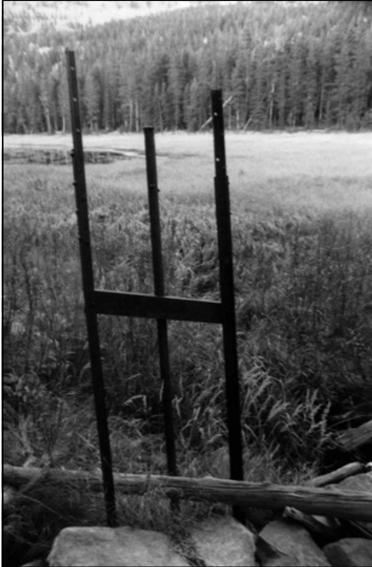
HAER UT-42-N. Water Lily Lake Dam. Headgate with lake in background; view to the north.
