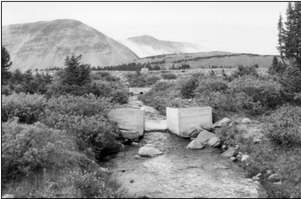
HAER UT-42-H. Five Point Lake Dam. Overview showing gauging box, check dam, looking upstream toward downstream outlet, dam, and control box; view to the west.
