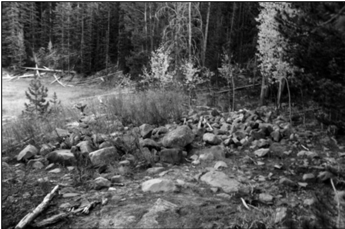
HAER UT-42-N. Water Lily Lake Dam. Rocks at south end of dam; view to the southeast.
