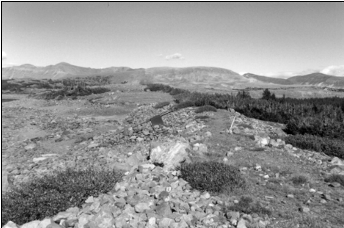
HAER UT-42-L. Superior Lake Dam. Overview of top of dam showing control box; view to the northeast.
