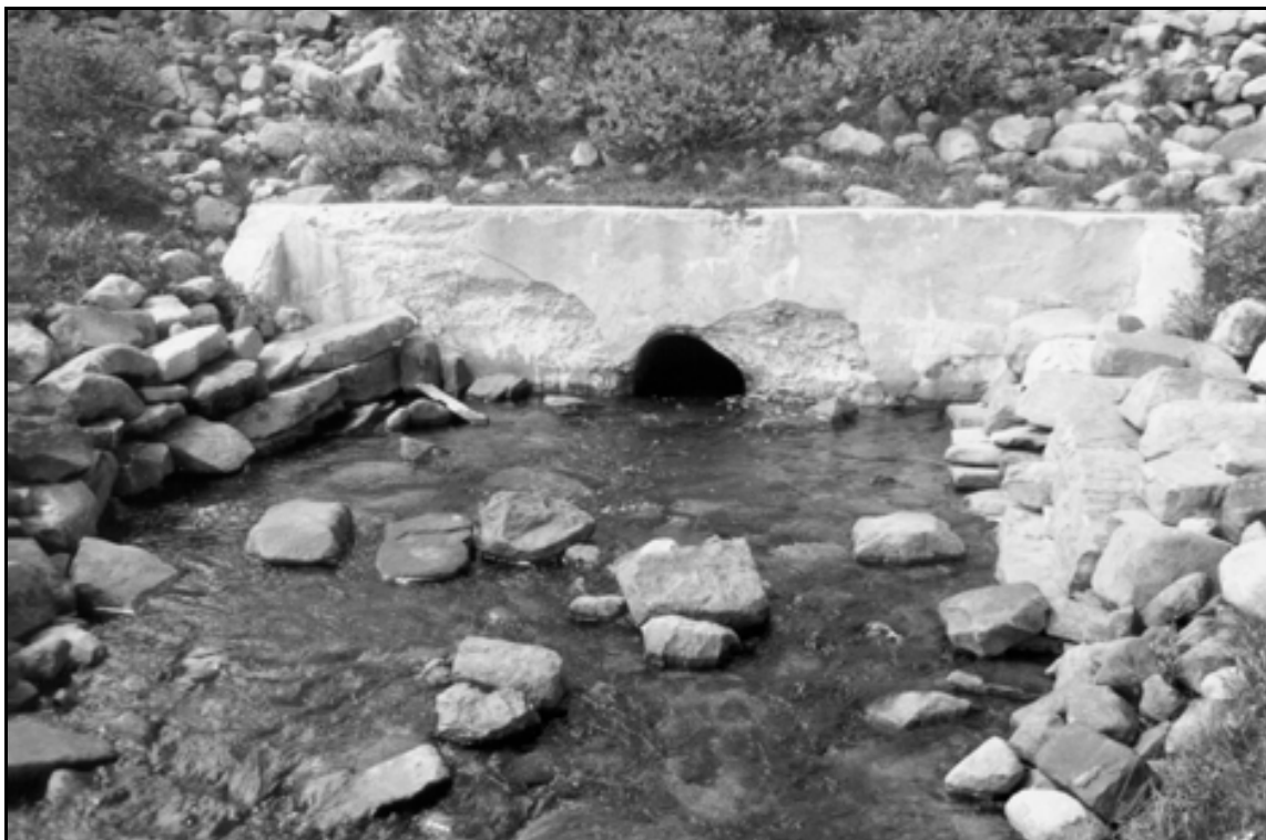
HAER UT-42-H. Five Point Lake Dam. Close-up view of downstream outlet; view to the west.
