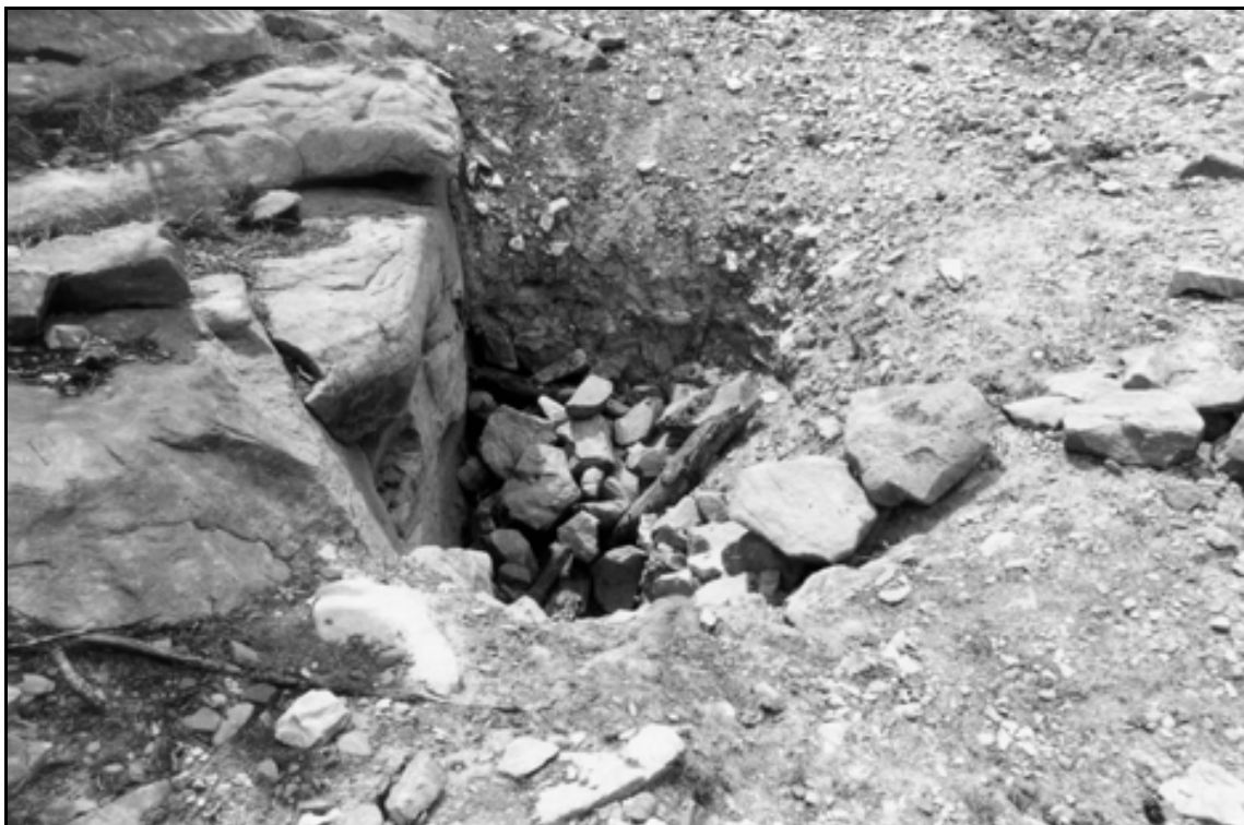
HAER UT-42-G. Farmers Lake Tunnel. Collapsed tunnel shaft; close-up view to the northwest.
