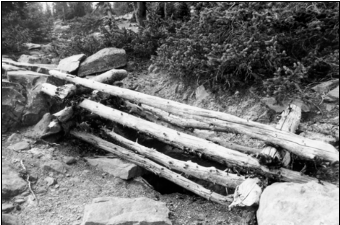
HAER UT-42-G. Farmers Lake Tunnel. View of cribbing over gate control shaft; view to the southwest.
