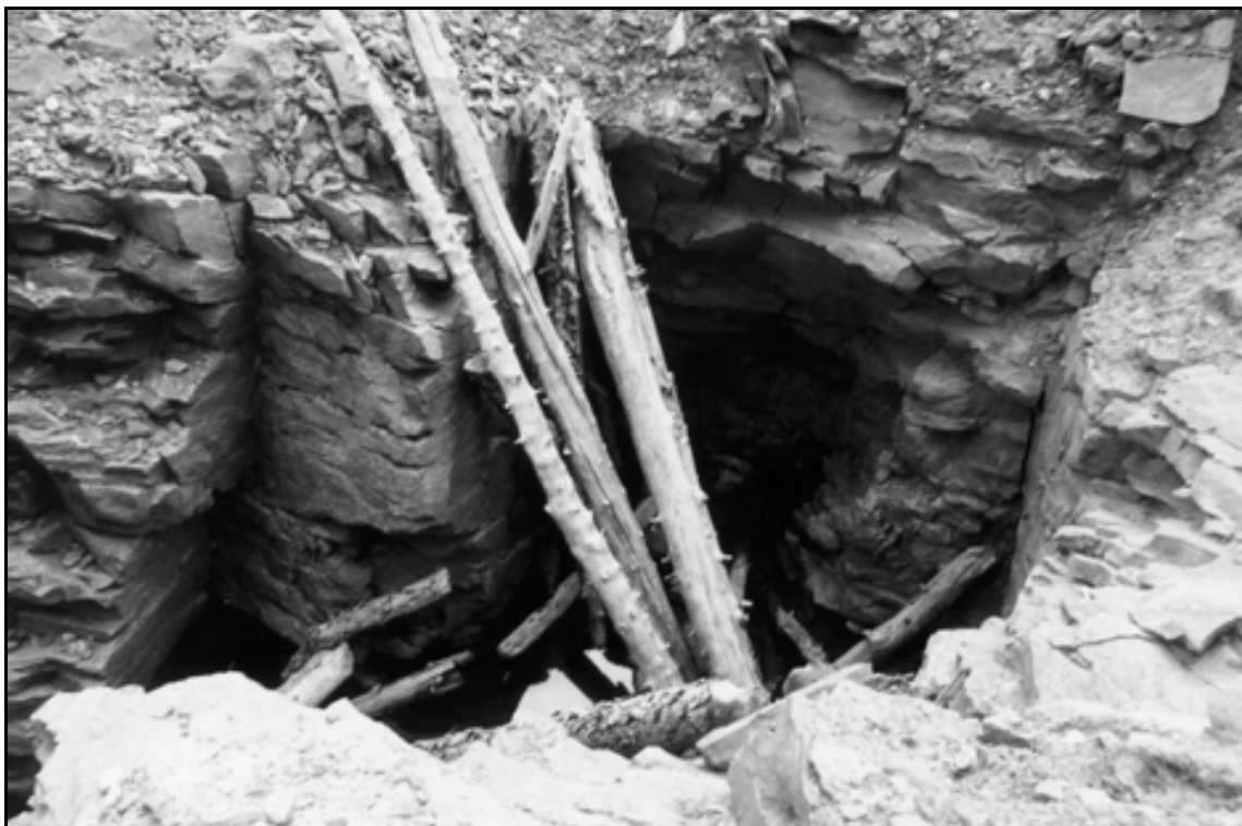
HAER UT-42-G. Farmers Lake Tunnel. View of the beginning of the tunnel inlet from above, showing remains of log grizzly; view to the southeast.
