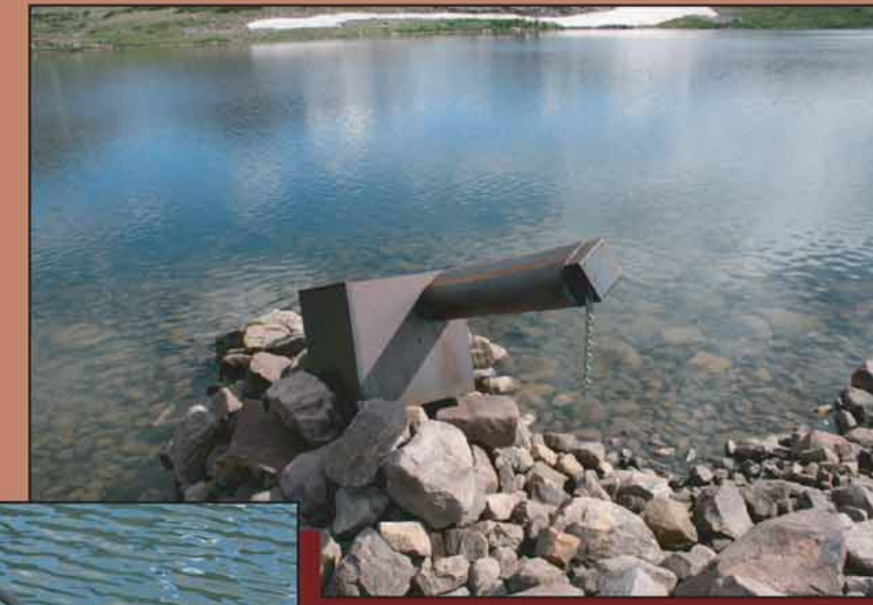
Top photo: Superior Lake headgate used to control water flow downstream.
