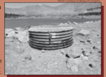
This steel downstream outlet valve at East Timothy Lake has been removed, but portions of the dam remain intact.
