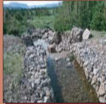
Superior Lake outlet with stone riprap to reinforce stream banks when large volumes of water were released downstream.
