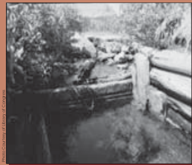
The log crib outlet at White Miller Lake was used to control water flow downstream. Note the stone reinforcements.
