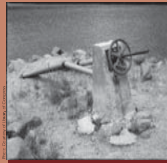
The headgate at Brown Duck Lake used to control the amount of water released downstream.
