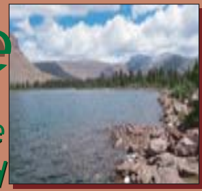
View of Farmers Lake from the upstream outlet channel.
