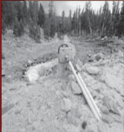
Outlet control gate on top of Island Lake dam regulating water flow downstream.
