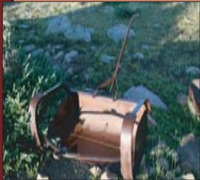
Drawn by horse cart, the Fresno Scraper moved and leveled large volumes of soil during dam construction.
