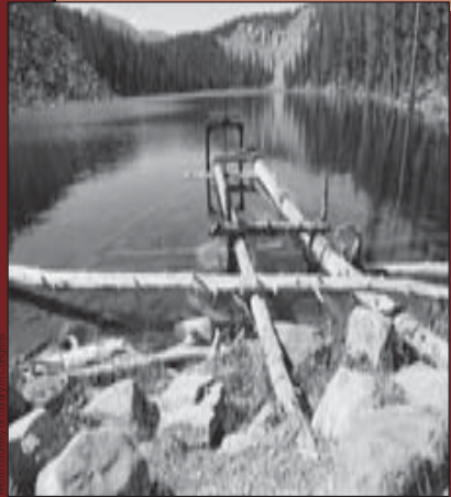
Headgate wheel above intake valve at Deer Lake used to regulate water flow downstream.
