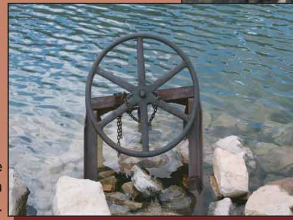
Drift Lake headgate. Note the different headgate styles between Drift and Superior Lakes.
