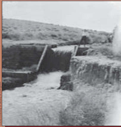
A wooden drop in the Dry Gulch Irrigation Canal diverting water from the Lake Fork River (ca. early 1900s)
