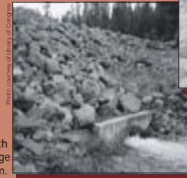
Top photo: Headgate used to control the amount of water released downstream at Island Lake.
