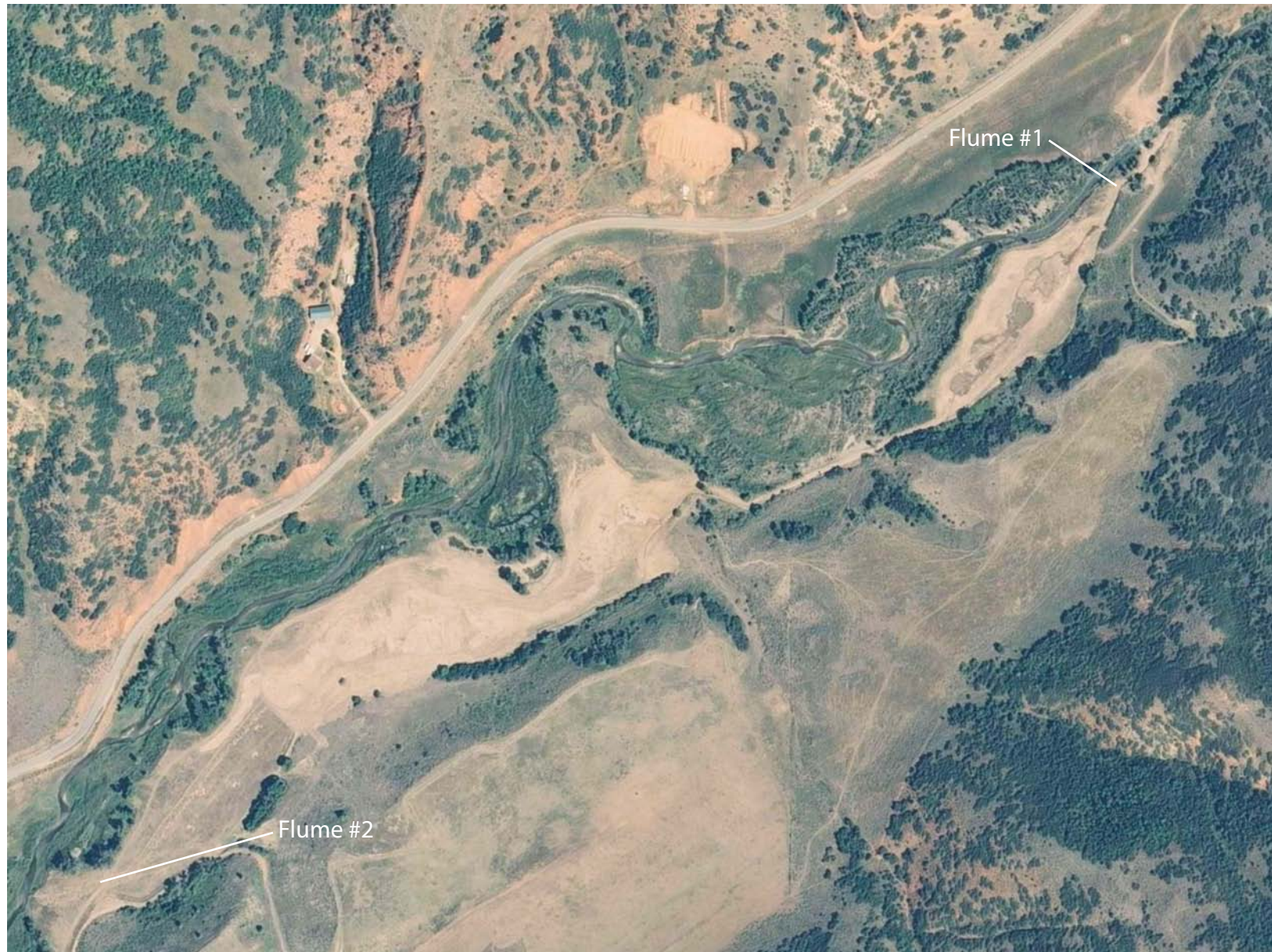
Figure 1. Aerial image taken in 2009, showing recently completed construction and location of two ramp flumes.
