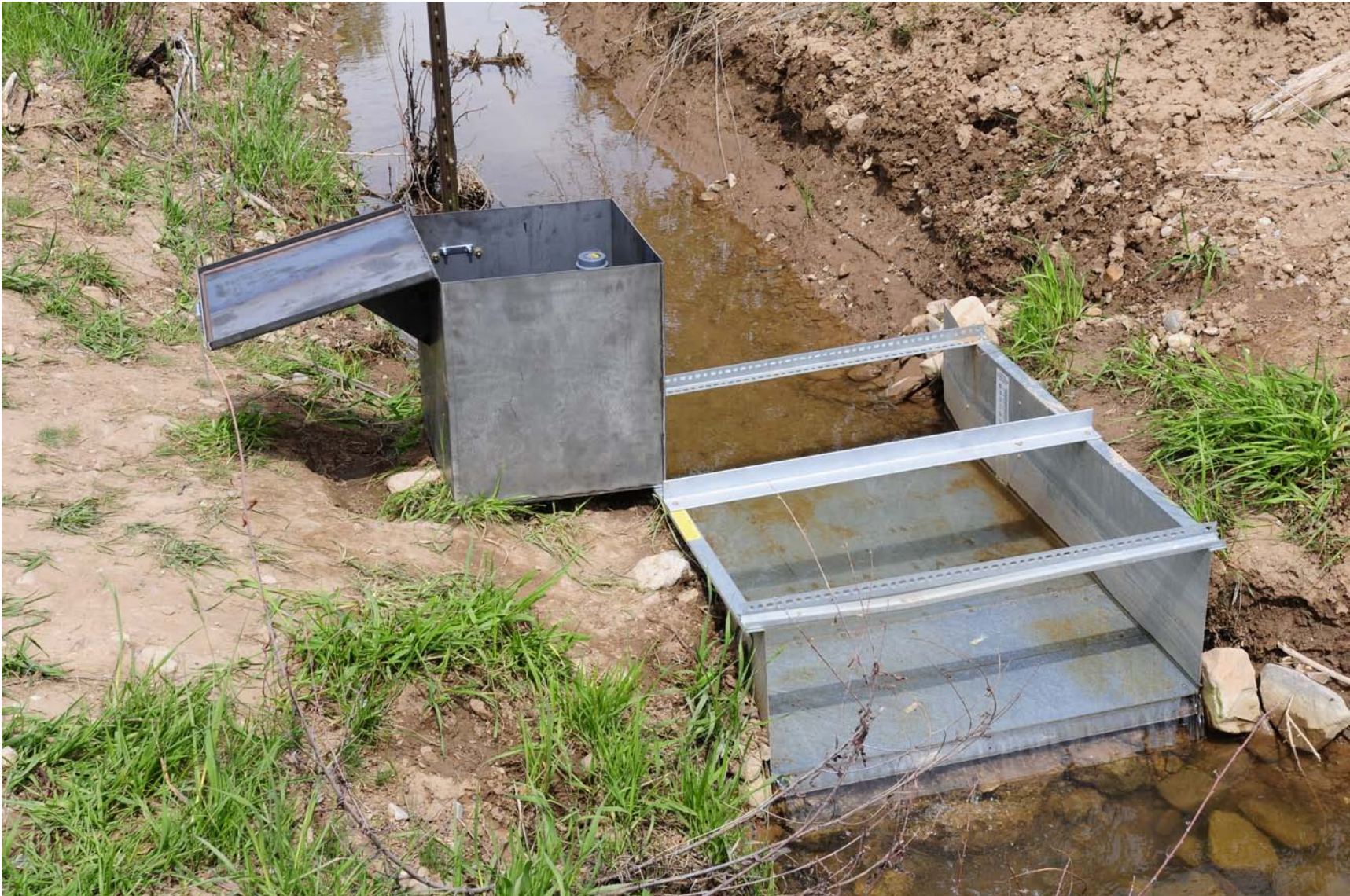
Figure 4. Lockable steel box that protects the instrumentation equipment. The lid and triangular support provide a sloping table for field computers.
