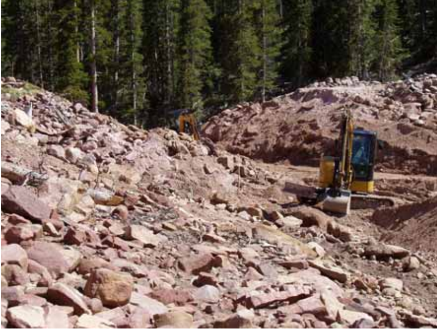
Figure 9: Crew using mini-excavator to cut through dam.
