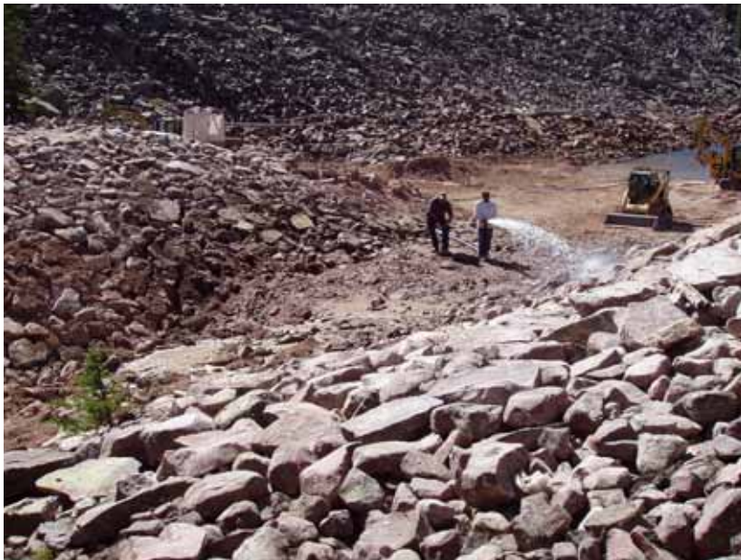
Figure 13: Crew washing fines into channel.
