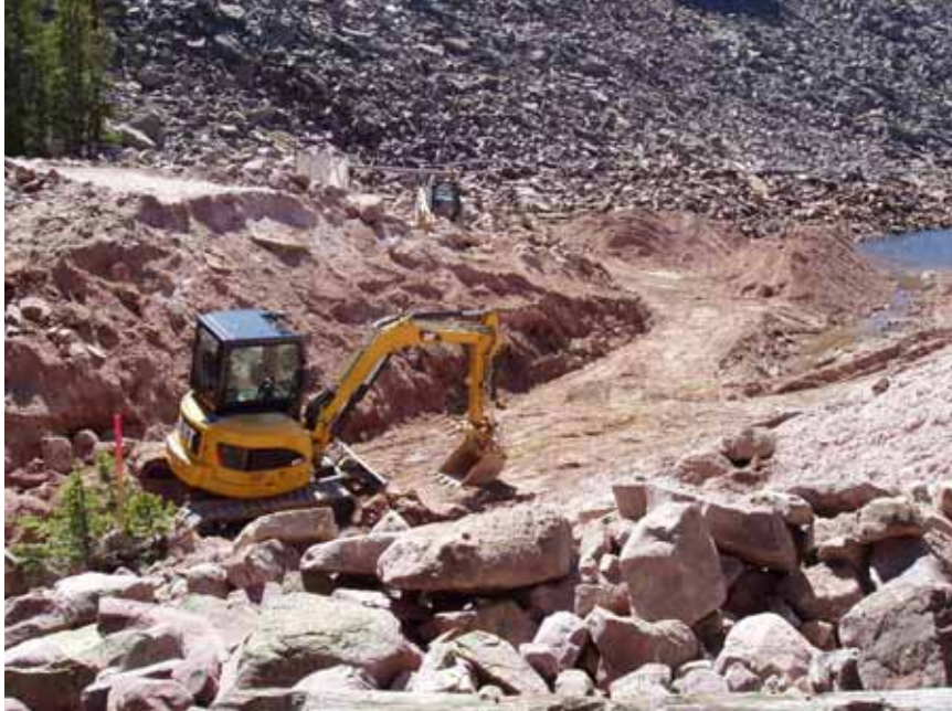
Figure 7: Crew excavating down to outlet pipe.
