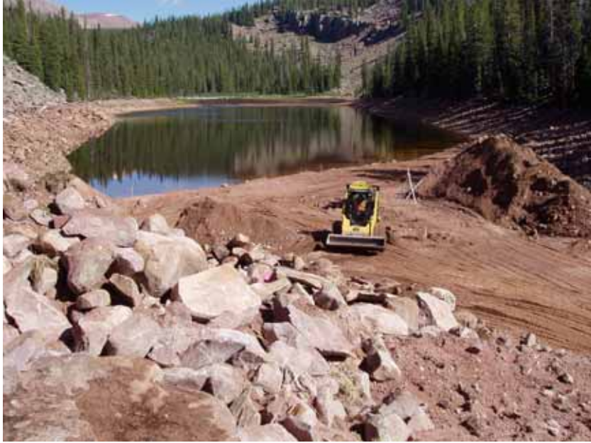
Figure 12: Looking upstream at the breach.
