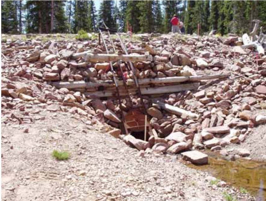
Figure 4: Deer Lake dam and head gate before removal.
