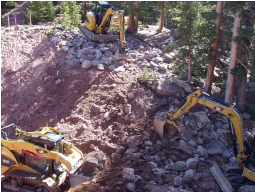
Figure 11: Reclamation crew placing riprap in breach.
