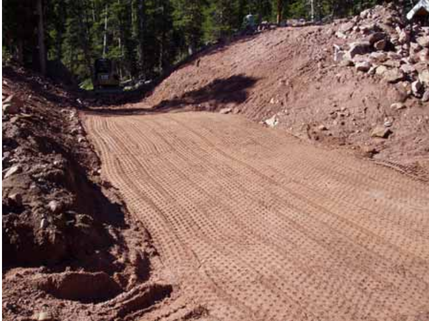
Figure 10: Looking downstream through the completed breach before riprap and rock sills were placed.
