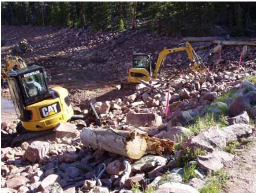
Figure 5: Reclamation crew using mini-excavators to remove riprap and cut breach through dam.
