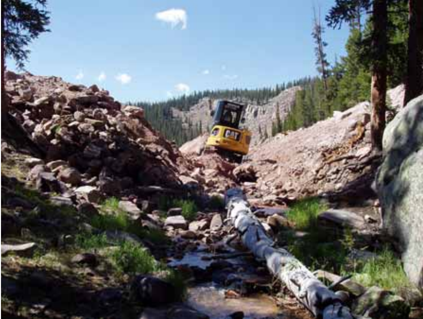
Figure 6: Crew continued cutting through Deer Lake dam – looking upstream.
