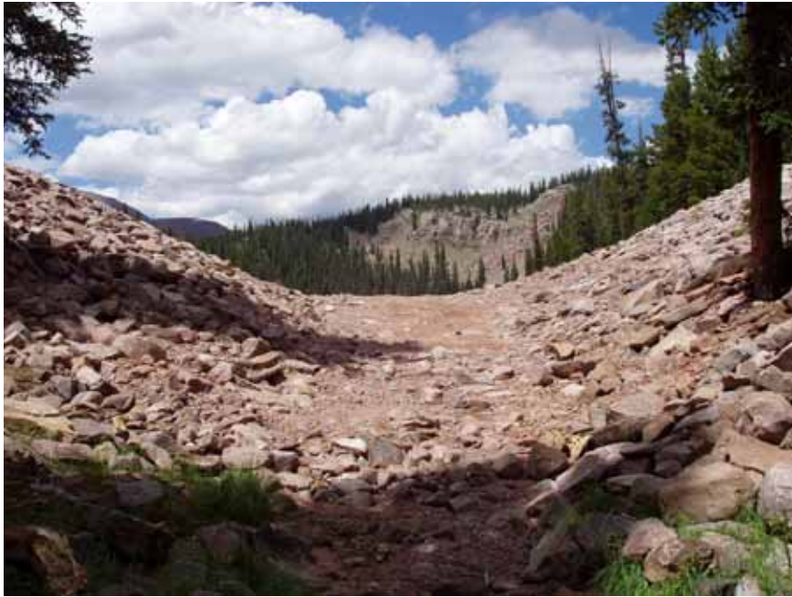
Figure 14: Looking upstream at the completed breach at Deer Lake.
