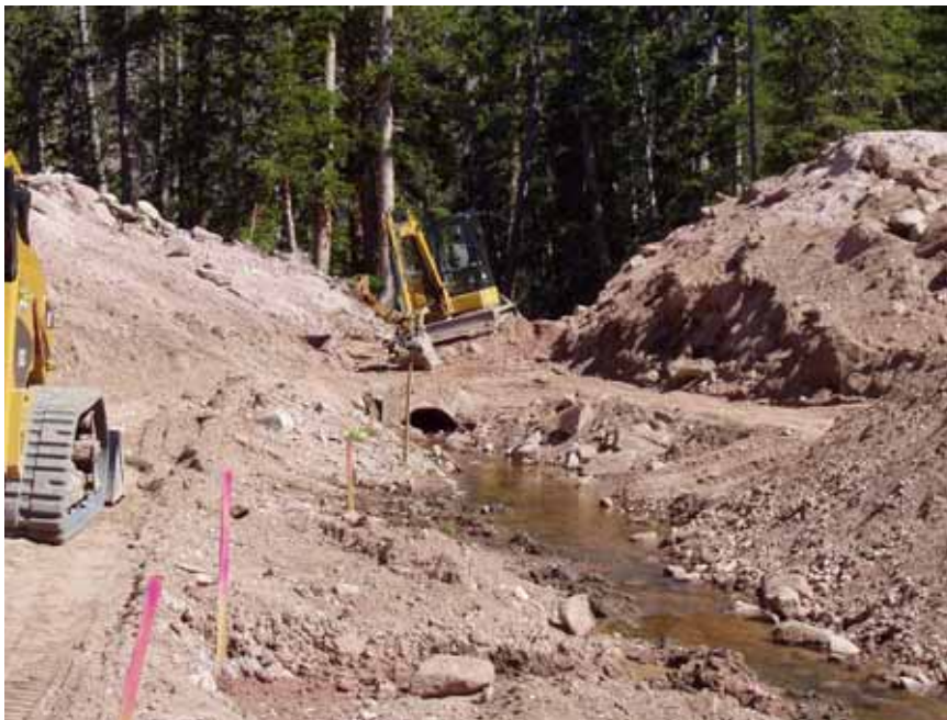
Figure 8: View of existing outlet pipe w/ breach cut through the dam.
