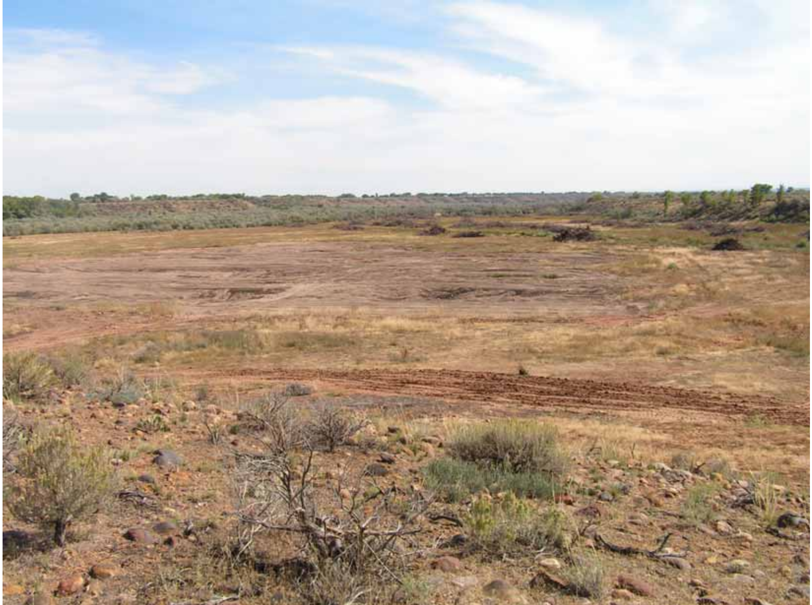
Figure 12. Photograph of the newly-constructed wetlands after application of the topsoil mixture.
