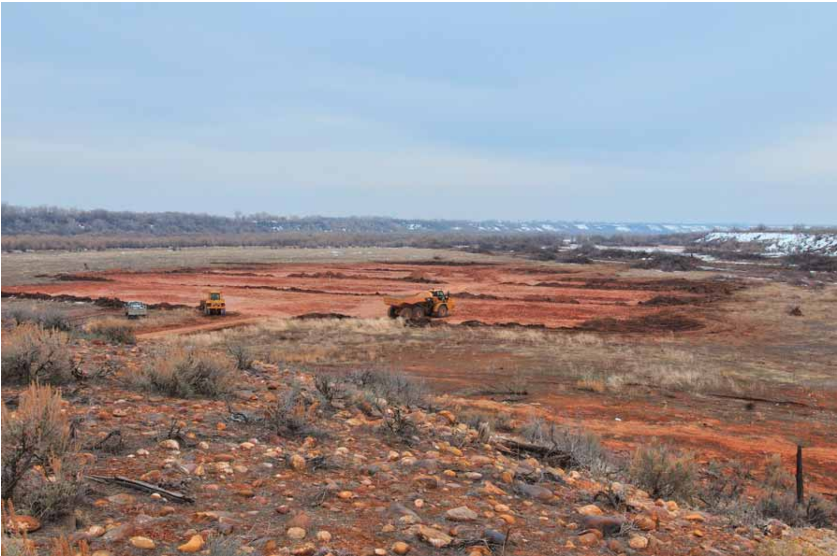
Figure 11. Photograph of the mitigation site taken in March 2008. The bulk of earth movement was mostly completed, but contouring, shaping, and topsoil application were still needed.
