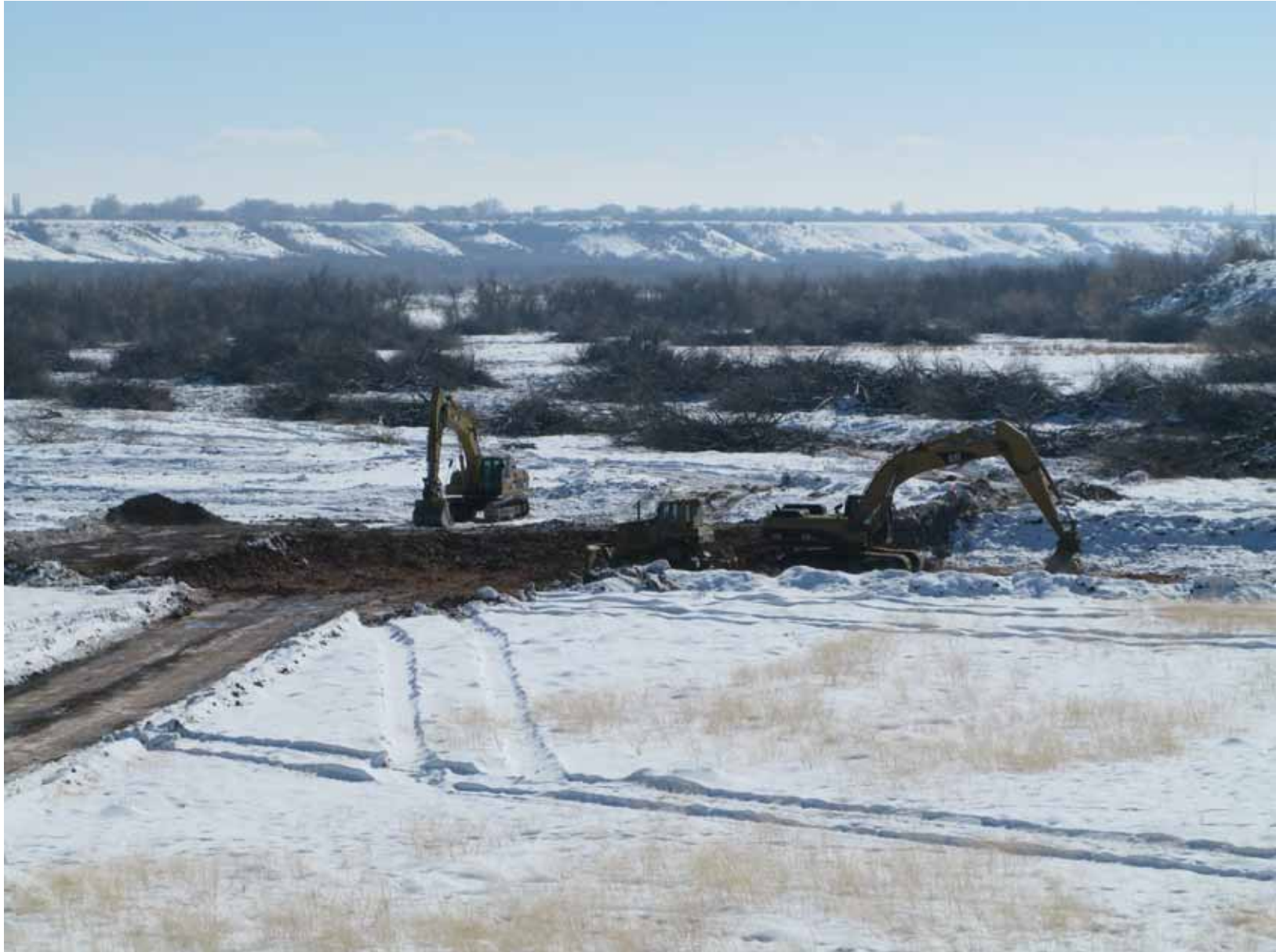
Figure 10. Photograph of the mitigation site following removal of Russian Olive trees. The trees have been uprooted and placed into piles for subsequent burning. This image also shows the beginning of wetland excavation.
